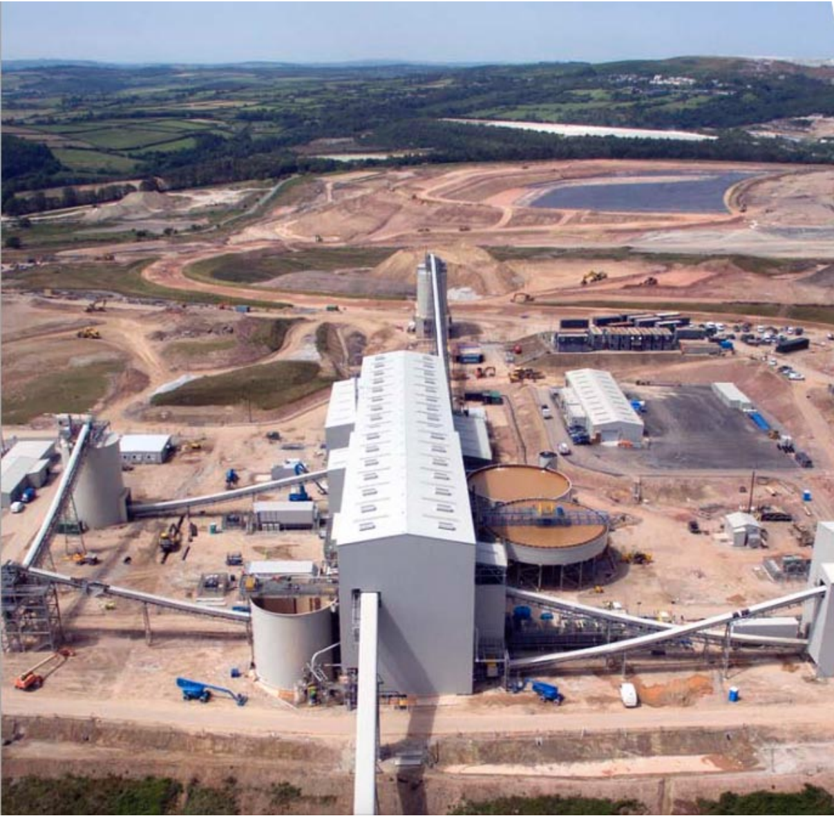
Figure 3: Drakelands tungsten ore processing plant and tailings pond/mine waste storage facility shortly after commencing production in mid-2015 near Plymouth in Devon, England
