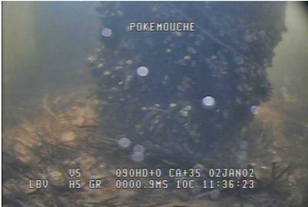
T3: Blue mussels on wooden column in the 20-25 m segment
