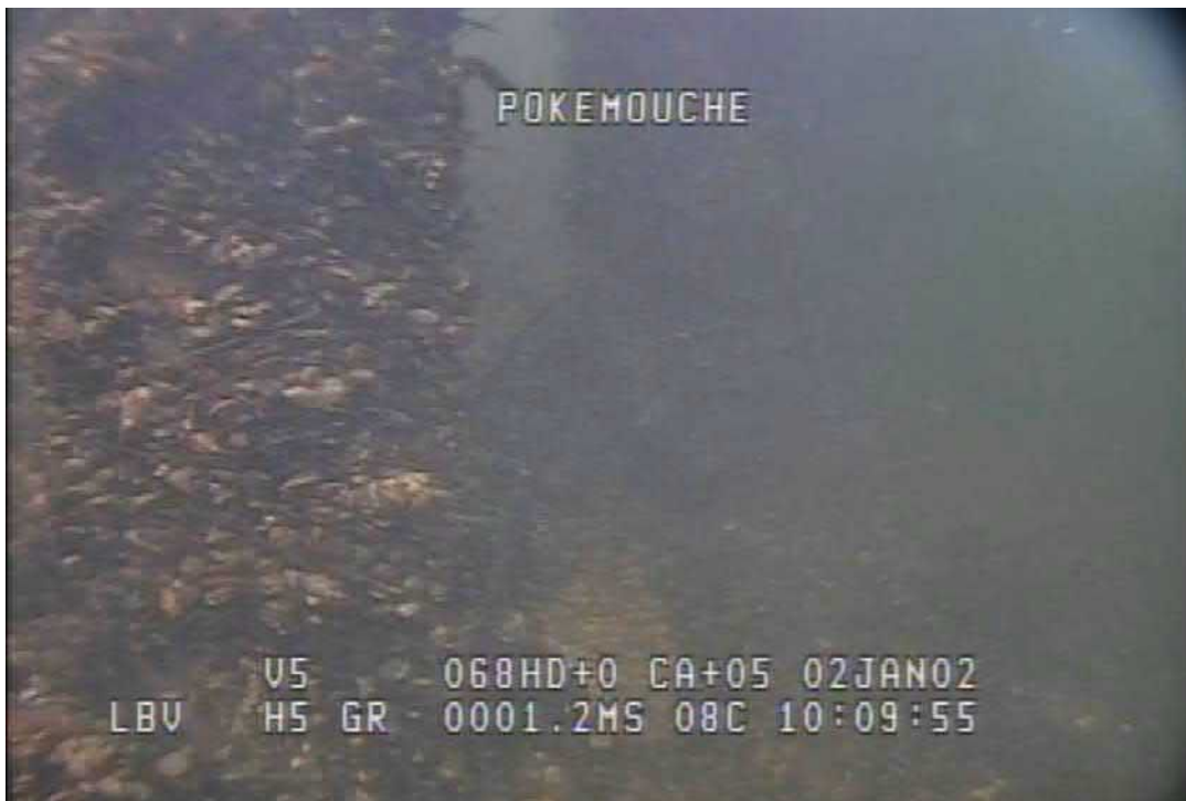
T6: Blue mussels on wooden column in the 15-20 m segment.
