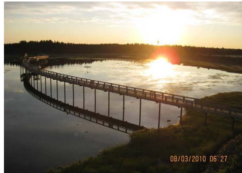
Receiving water in impoundment
