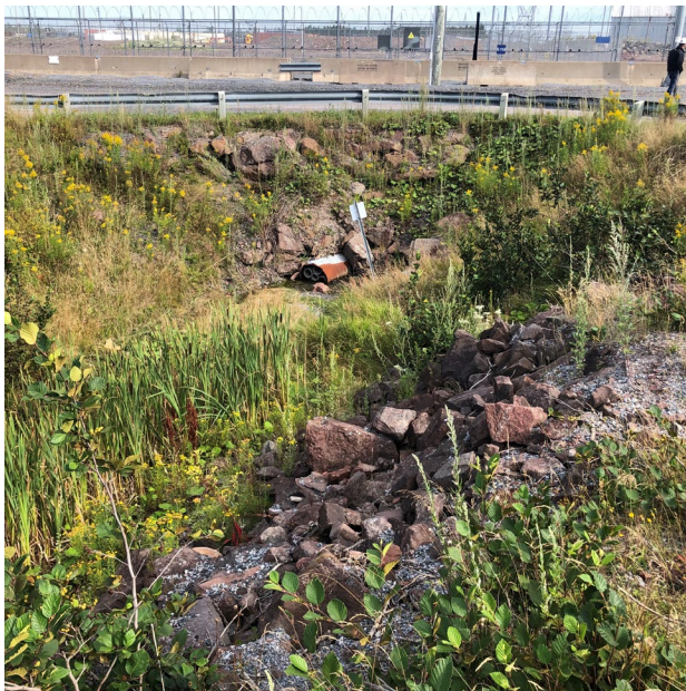
Photo 7 View of Northern Extent of Drainage Channel, Looking North (August 16, 2022)
