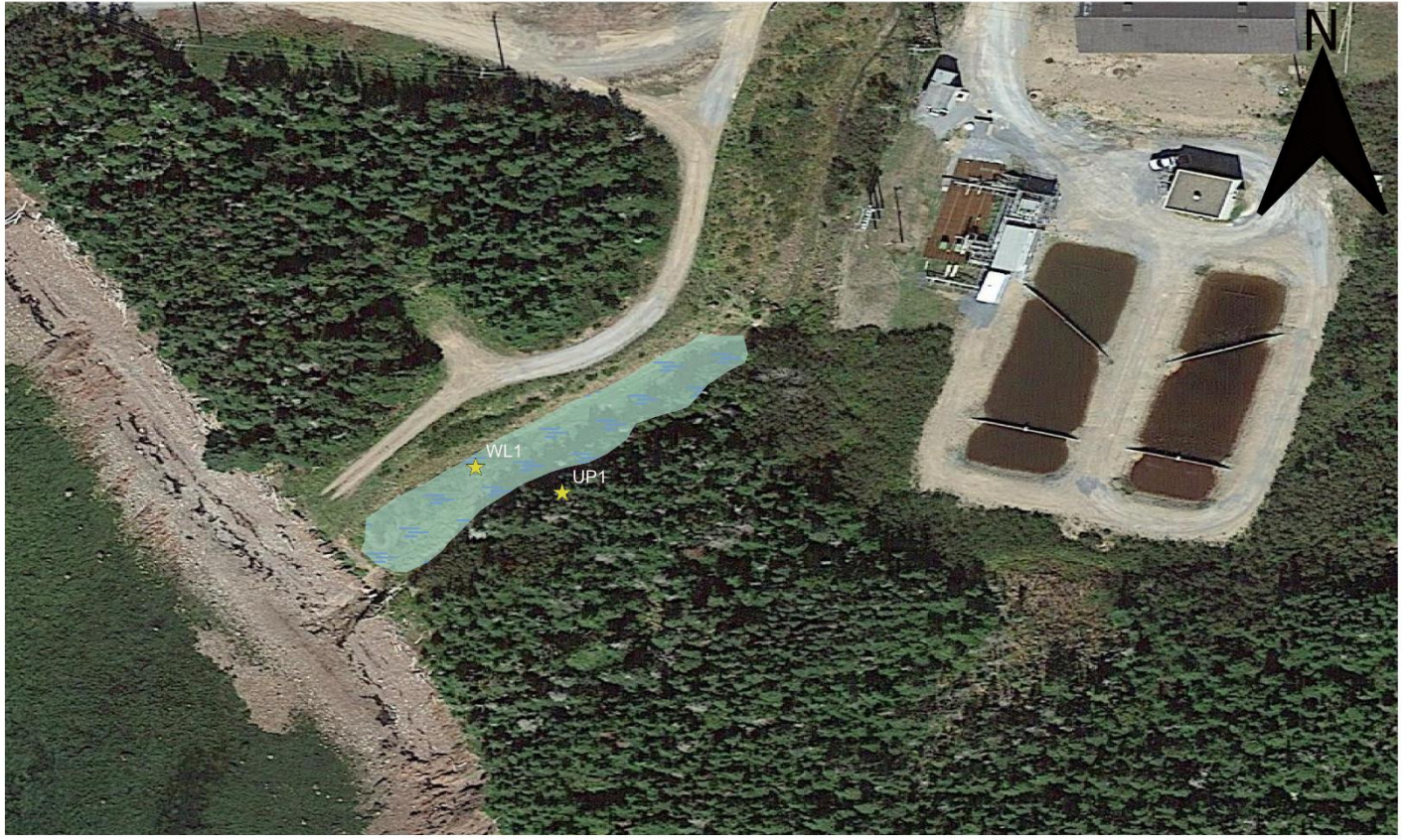
Figure 1 – Wetland and plot points for NB Power Nuclear Generating Station Domestic Sewage Treatment Plant Upgrade
