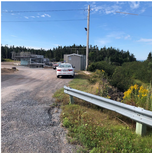
Photo 3 View of Project Area, Looking South (August 16, 2022)
