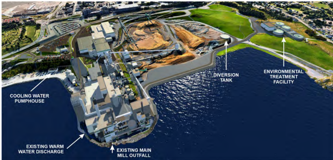
Figure 20. Major components of the environmental treatment facility and water use reduction project proposed for the Reversing Falls Mill in Saint John, New Brunswick.
