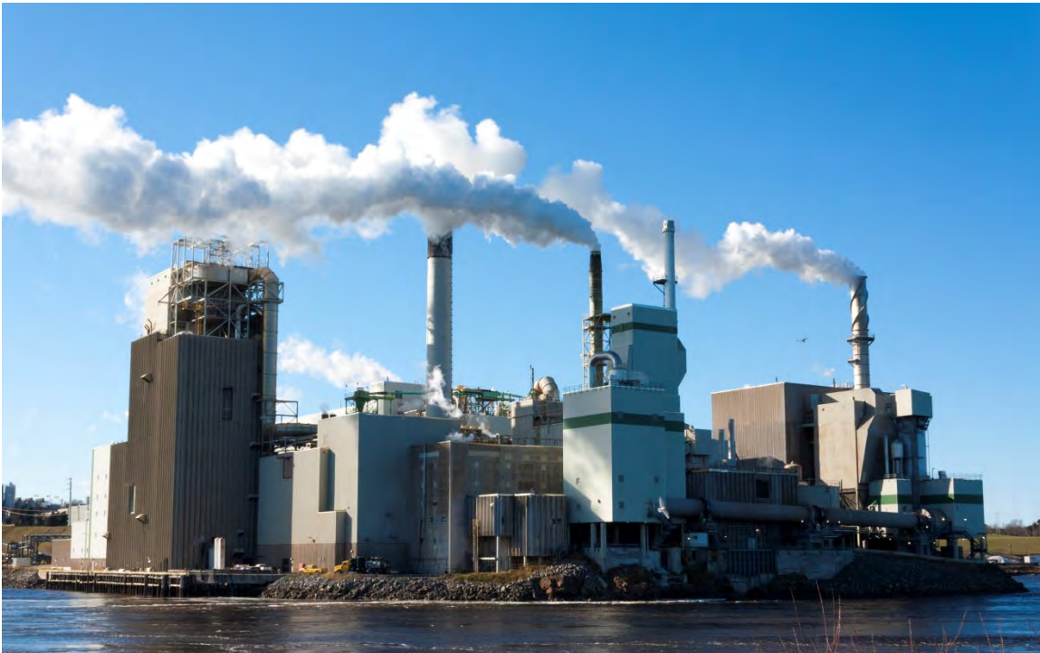
Figure 2. The Reversing Falls Mill located near the mouth of the Saint John River in Saint John, New Brunswick.
