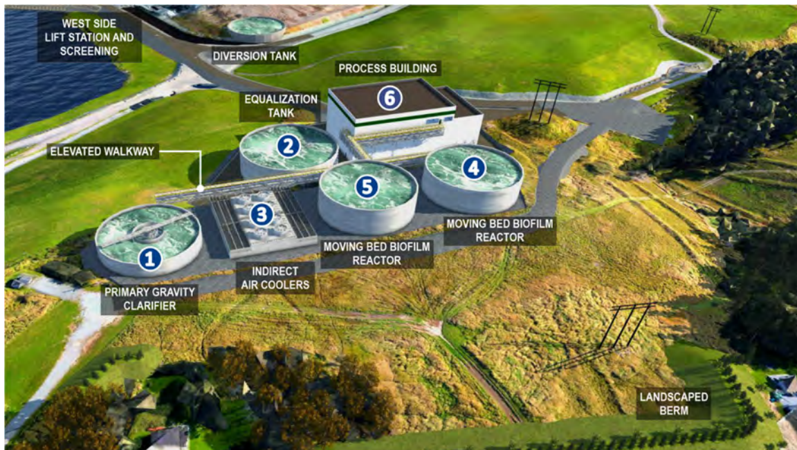
Figure 21. General layout and main components of the environmental treatment facility proposed for the Reversing Falls Mill in Saint John, New Brunswick. The numbers follow the effluent through the treatment process.
