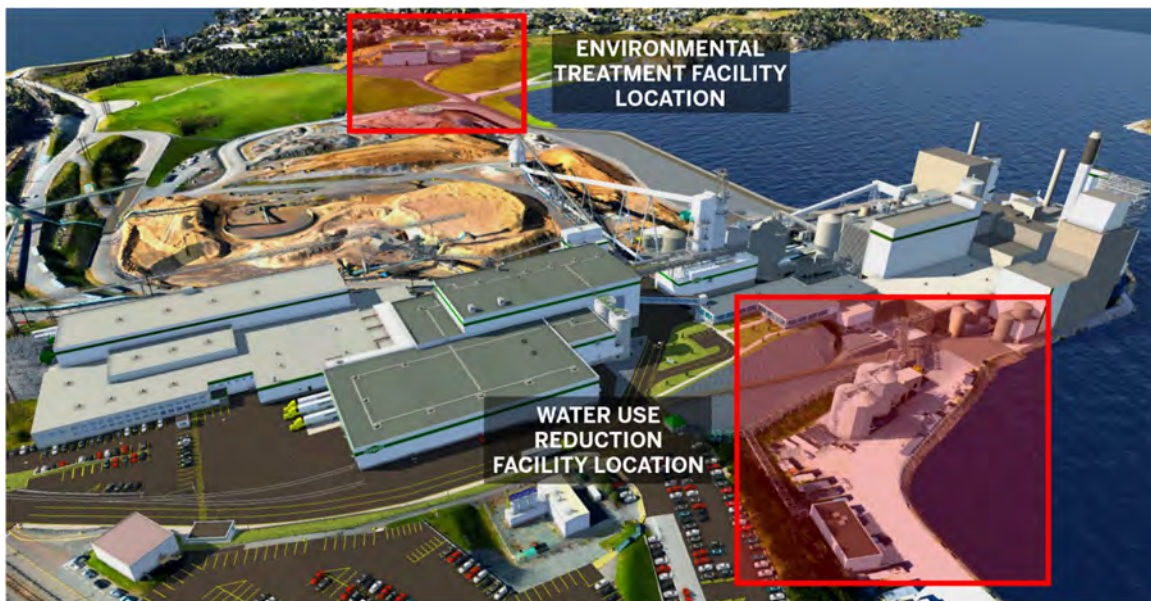
Figure 5. Oblique view showing the general location of the environmental treatment facility and the water use reduction infrastructure ( i.e. , shown within red boxes) proposed for the Reversing Falls Mill in Saint John, New Brunswick.
