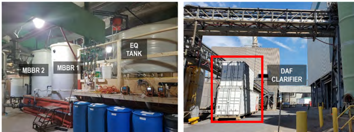
Figure 17. Photograph showing the moving bed biofilm reactor pilot plant that was operated at the Reversing Falls Mill in Saint John, New Brunswick.
