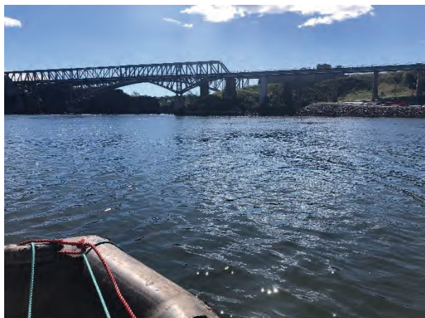
Photo 11: View of Downstream for 2.5 Hour Before High Tide Temperature Monitoring.
