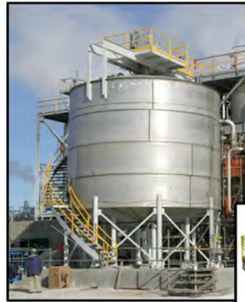
26' Clarifier Installation
