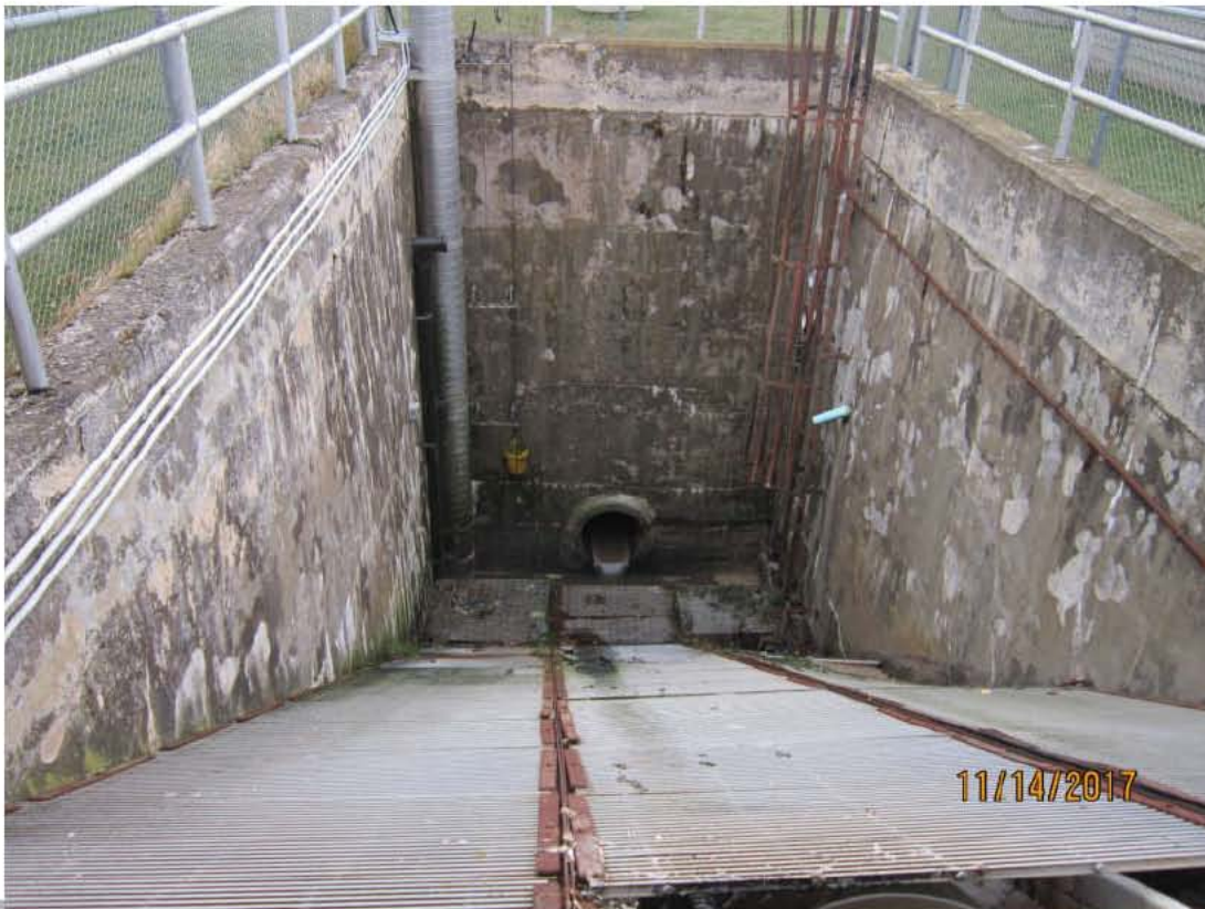
Figure 4: Screw Pump Wet-Well
