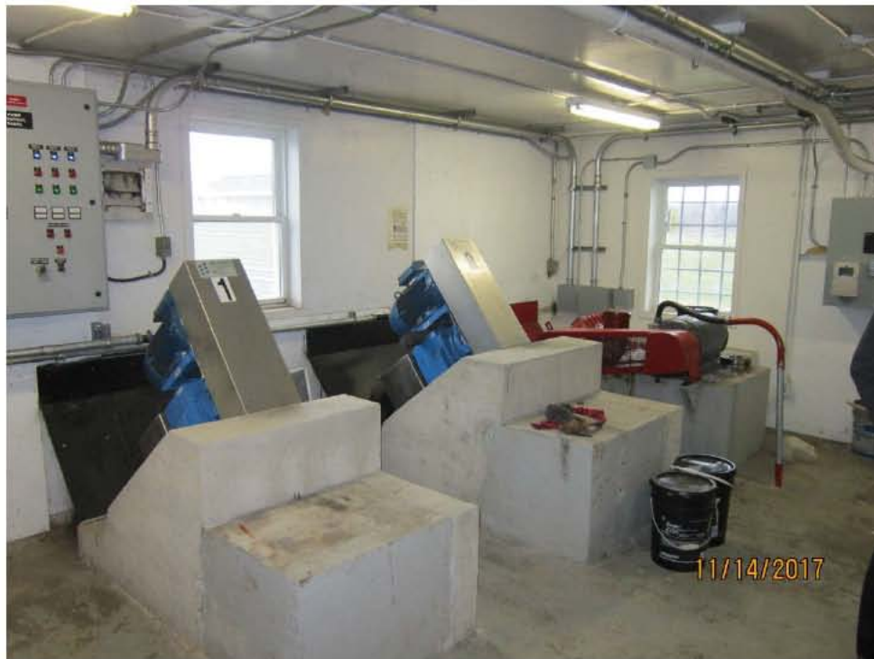
Figure 2: Screw Pump Motors and Mounting
