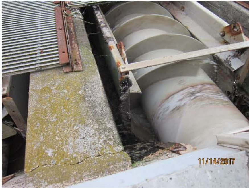
Figure 4: Screw Pump Wet-Well
