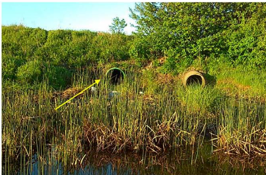
Shediac WWTP outfall
