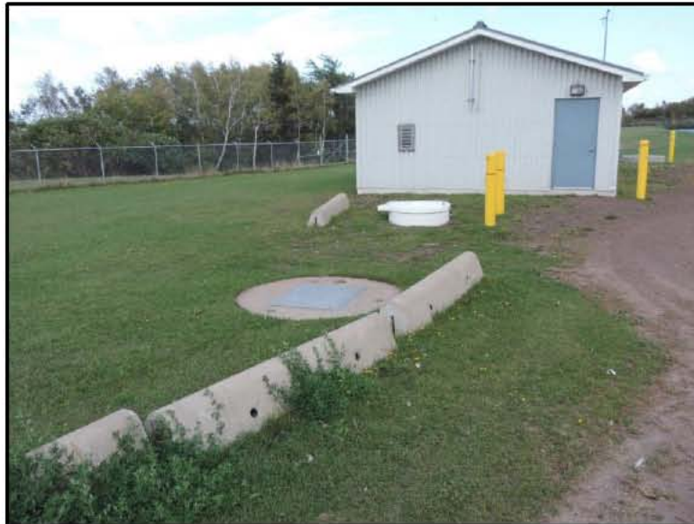
Photo 10 - Looking east towards the UV Treatment Building, which is located at the northeast corner of the existing Polishing Cell.
