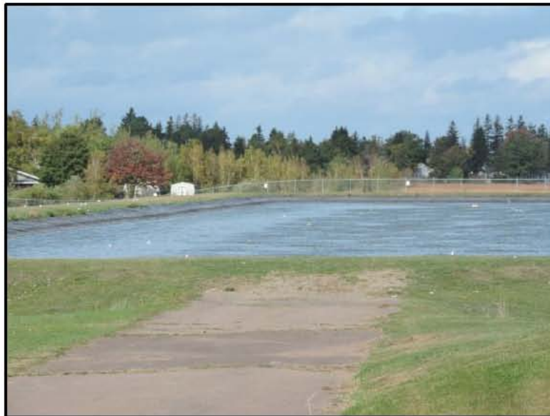
Photo 6 - View NNW to Aerated Lagoon No. 1, note residences in the left side of the photo.
