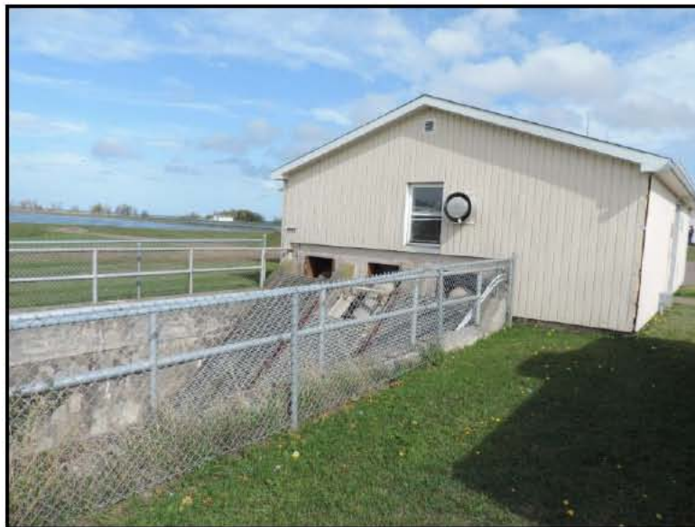
Photo 2 - The existing Screw Pump Building looking northeast.
