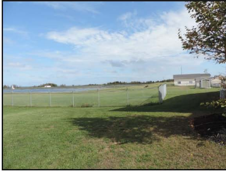
Photo 3 - View east with the lagoons to the left and the Pre-treatment Building closest to the fence and the Screw Pump Building to the extreme right. Photo taken from Cap-Brule Road.
