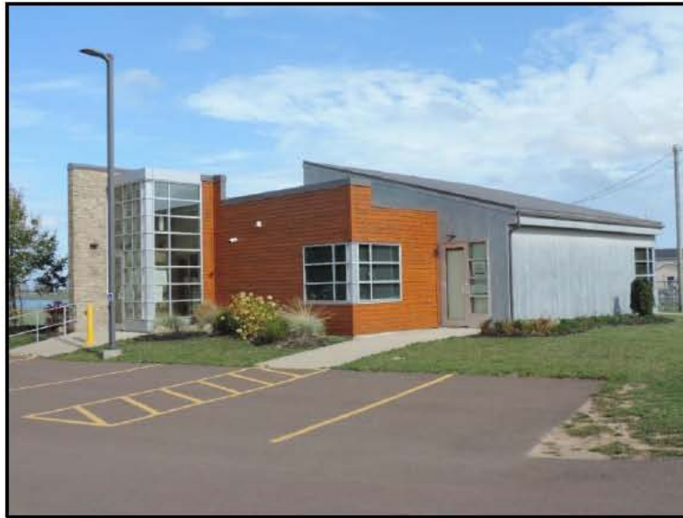
Photo 1 - View of the GSSC main office building looking northeast.
