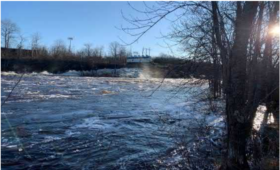
Photo 2 – Looking at the U.S.A. side in a south east direction below the Milltown Station (December 2020).
