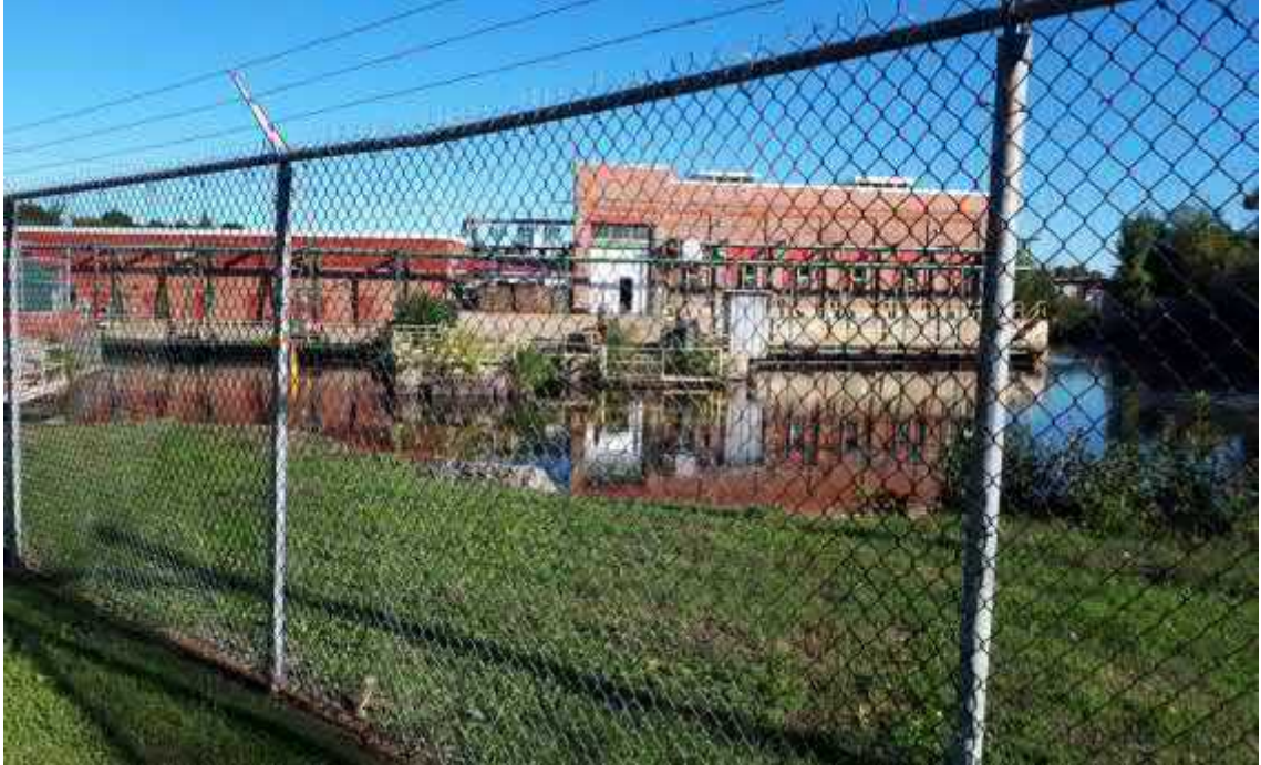
Photo 1 - Looking north at the Milltown Station from land above it (August 2020).
