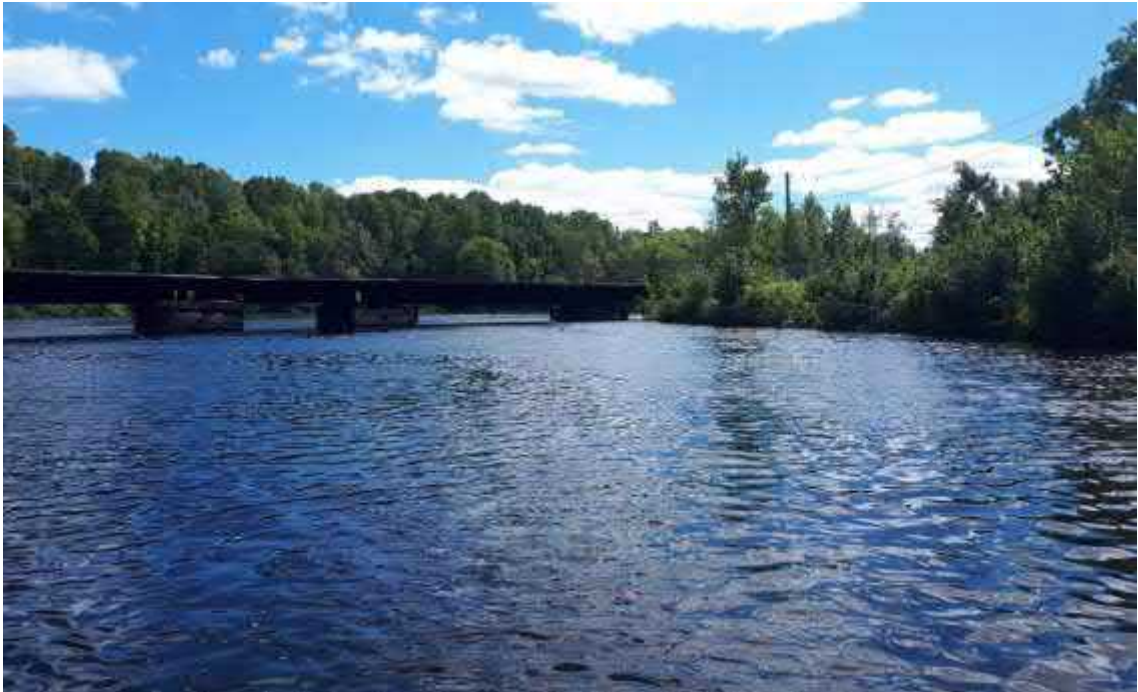
Photo 8 – Looking south at the train bridge just above the Milltown Station (September 2020).
