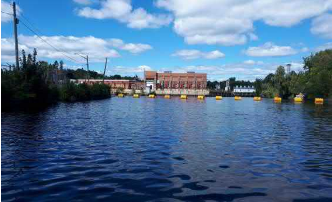
Photo 7 – Looking northwest at the Milltown Station from the water above it (September 2020).
