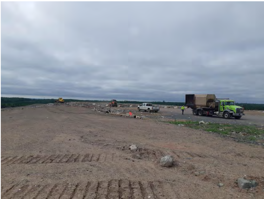
Photo 2: View of active landfill disposal cells in Area E (July 2, 2020).
