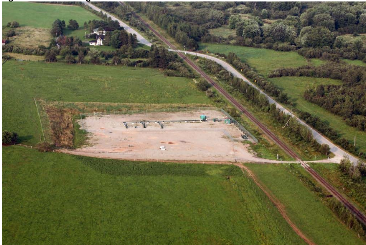
Figure 4.2 Existing F-67 Well Pad
