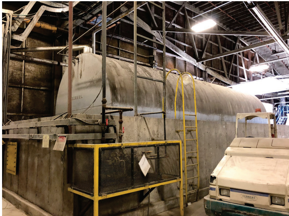
Photo 30 - View of 113,500L Furnace oil tank in north warehouse.
