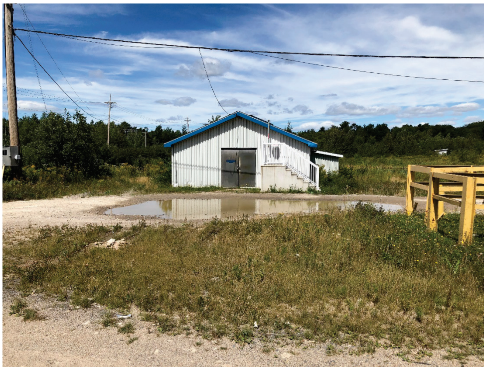
Photo 42 - View of fire pump house, looking north.
