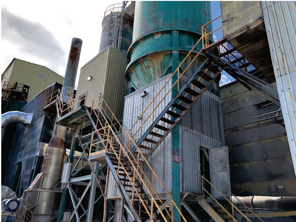
Photo 8 - View of calcine baghouse, looking southwest.
