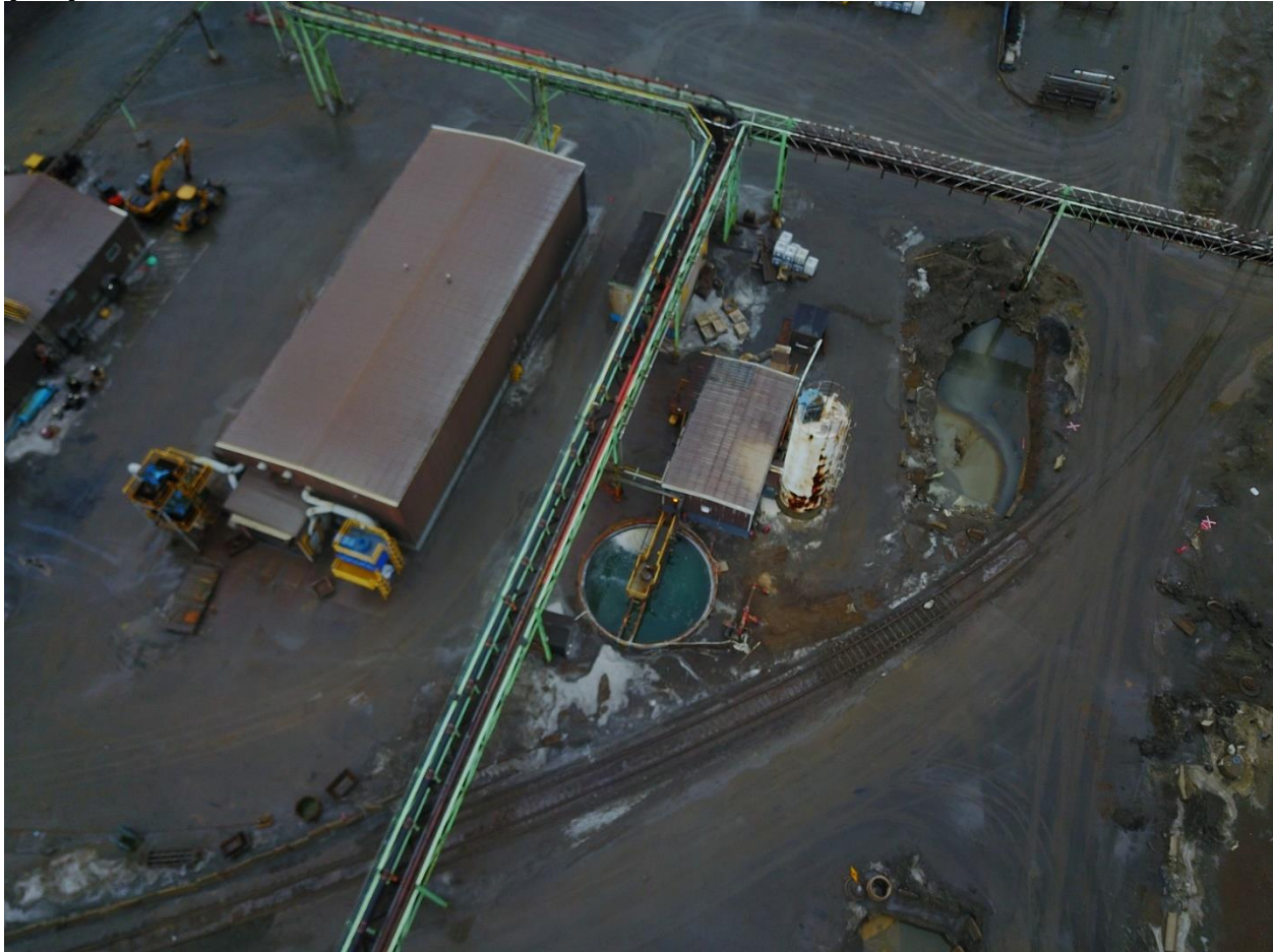
WWTP, CLARIFIER AND BRICK SHOP
