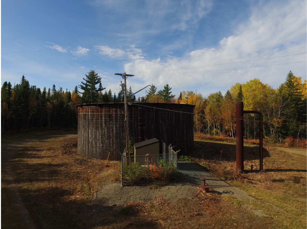
FRESH WATER RESERVOIR
