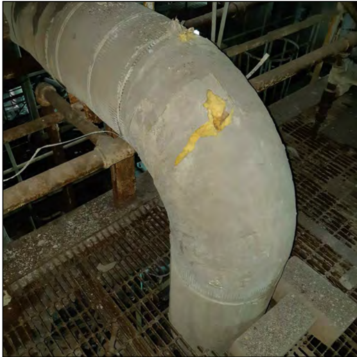
PHOTO 25 - LOCATION OF ACM SAMPLE 19ACM-3
