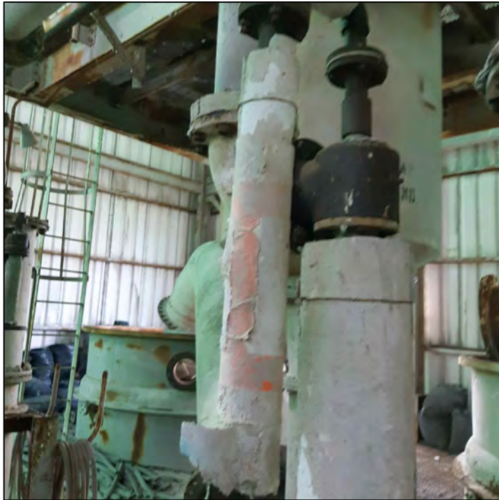
PHOTO 26 - LOCATION OF ACM SAMPLES 19ACM-5 AND 19ACM-6
