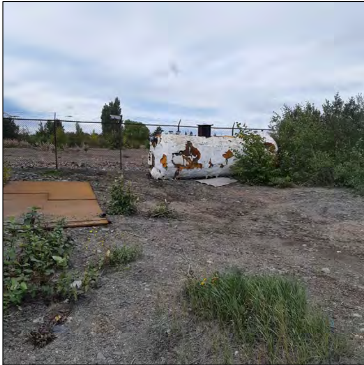
PHOTO 30 - LOCATION OF ACM SAMPLE 19ACM-10
