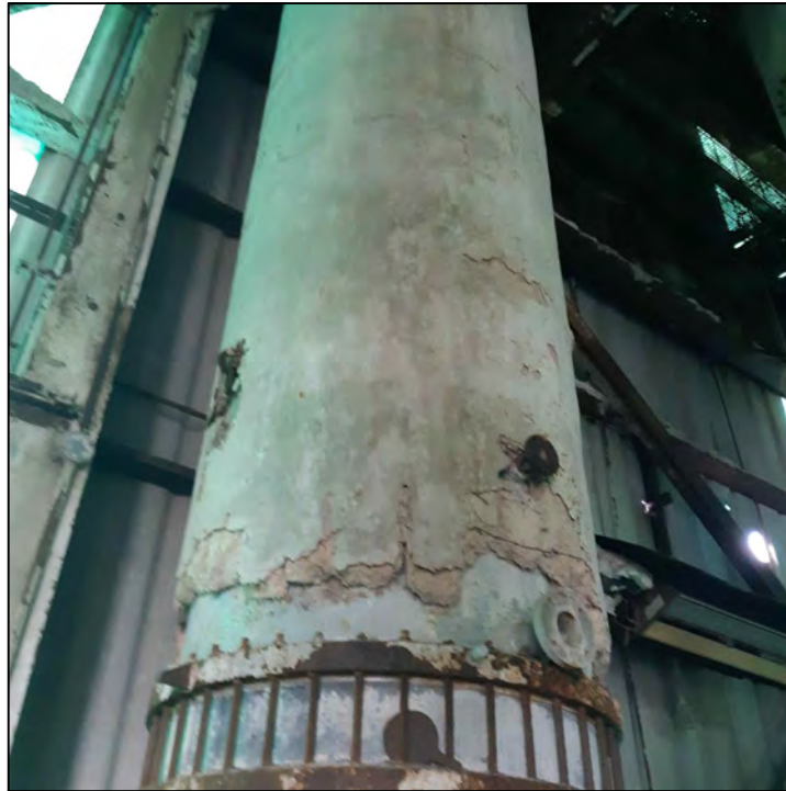
PHOTO 23 - LOCATION OF ACM SAMPLE 19ACM-1
