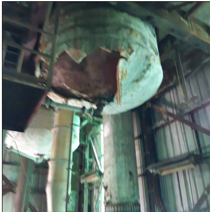
PHOTO 24 - LOCATION OF ACM SAMPLE 19ACM-2
