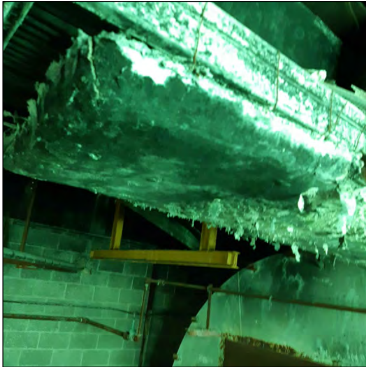
PHOTO 28 - LOCATION OF ACM SAMPLE 19ACM-8
