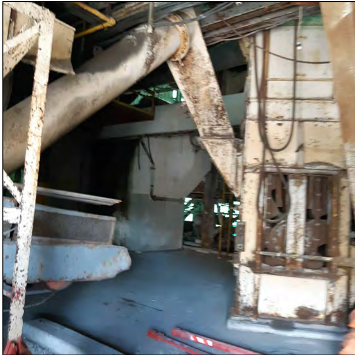
PHOTO 16 - MAIN FLOOR OF THE DAP BUILDING
