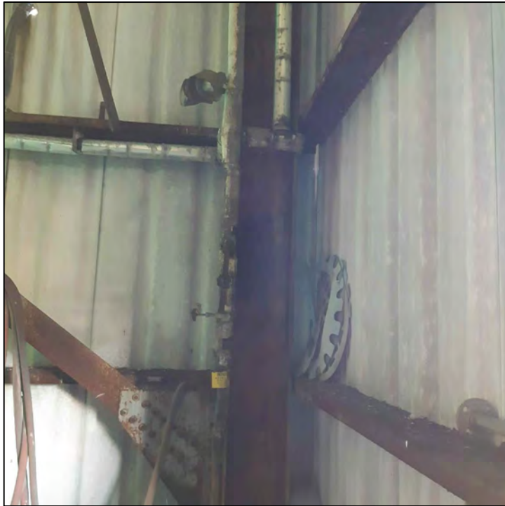
PHOTO 27 - LOCATION OF ACM SAMPLE 19ACM-7
