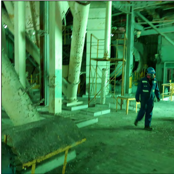
PHOTO 19 - 3RD FLOOR OF THE DAP BUILDING
