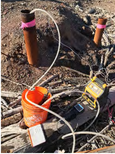
Photo #13: View of groundwater monitoring and purging equipment set up at existing monitor wells 05GW-30 (A, B and C).
