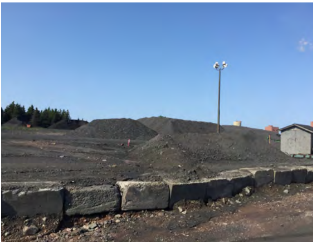
Photo #51: View of the Coke Fines Storage Area.
