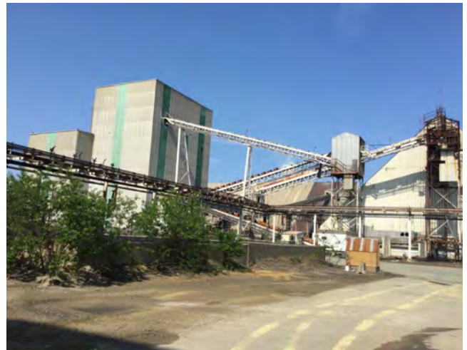
Photo #36: View of Conveyors at rear of DAP Building (Typ.).
