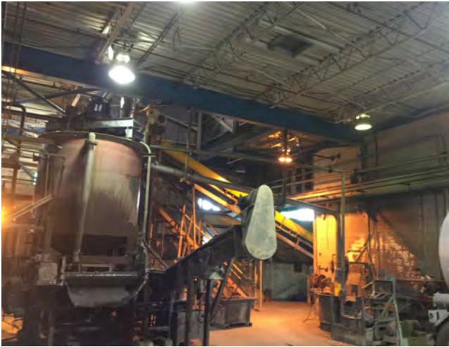
Photo #43: Inside view of the Battery Recycling Plant.
