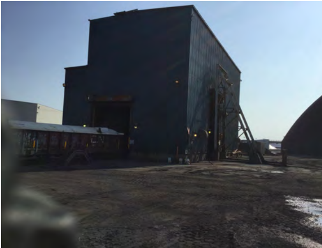
Photo #49: View of the Railcar and Truck Unloading Building.
