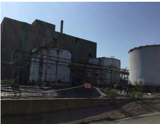
Photo #47: View of the Acid Process Tanks (three of the four).
