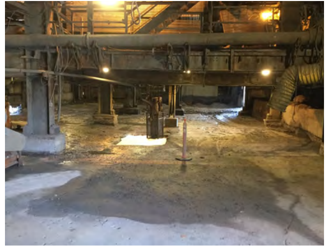
Photo #14: Bottom of the Crusher Building.
