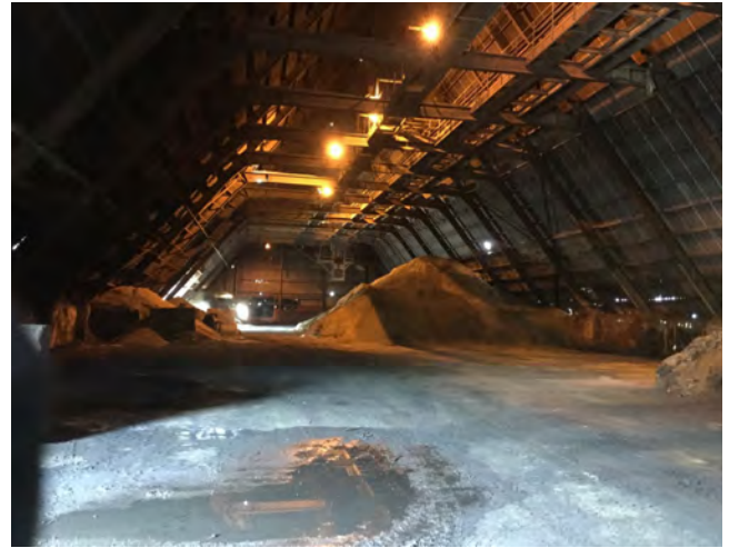
Photo #26: Inside view of the RMS Building.
