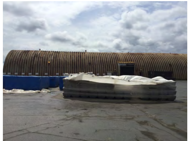
Photo #24: View of the Metal Quonset Building.
