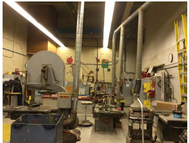
Photo #46: Inside view of the Carpenter Shop.
