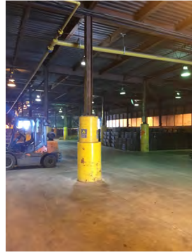
Photo #8: Inside view of the Metal Storage Building.
