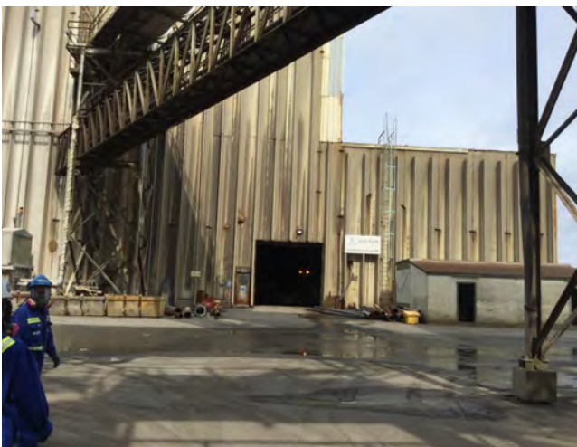
Photo #17: View of the Acid Plant.
