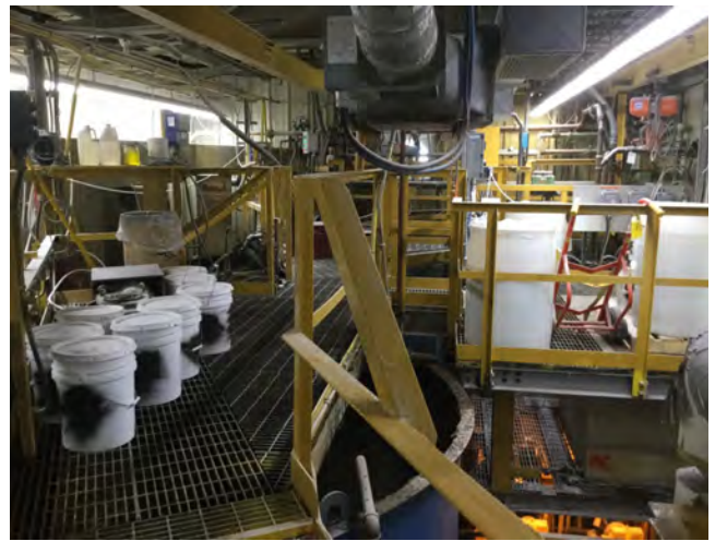
Photo #34: Inside view of the WWTP.
