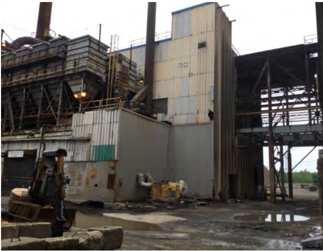
Photo #1: Looking at SRF Building from inside the Refinery.
