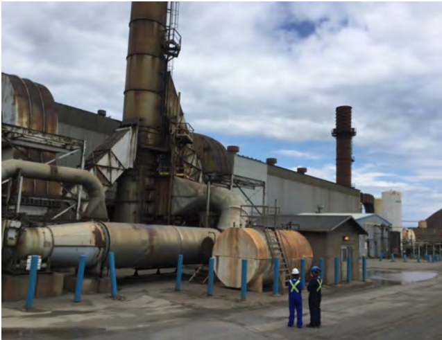
Photo #21: Front view of plant with Sinter Baghouse and Furnace Baghouse.
