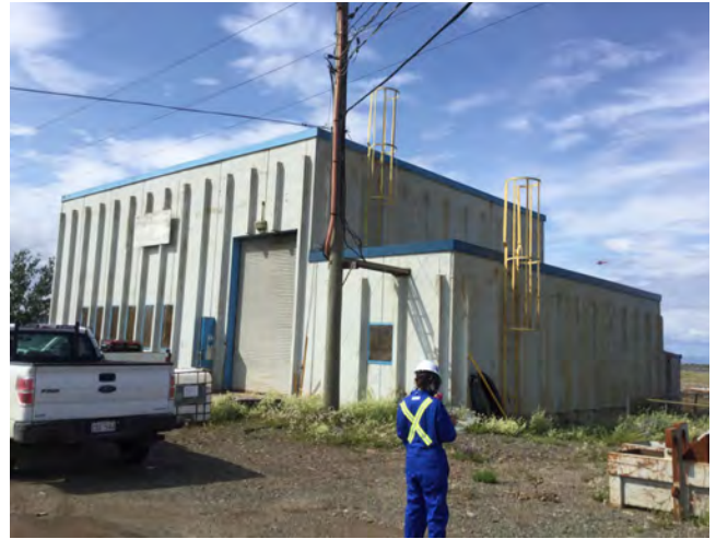
Photo #38: View of the Salt Water Pumphouse.
