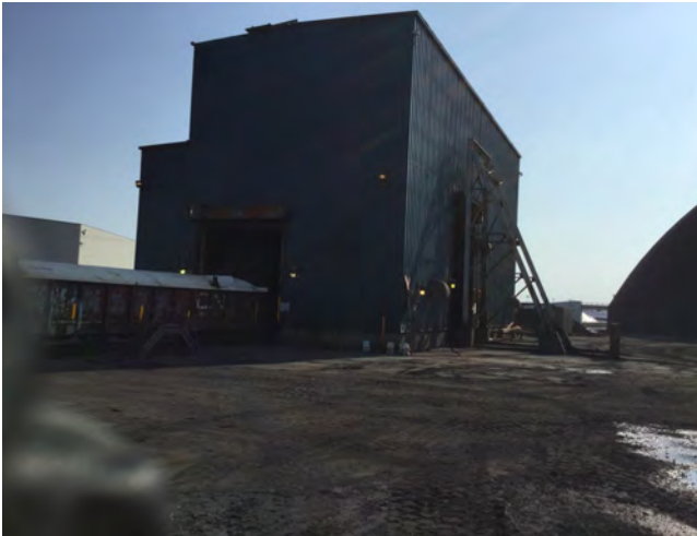
Photo #27: View of the Car Unloading Building.
