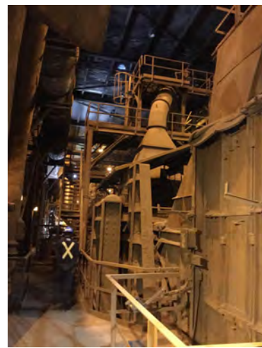
Photo #10: View of the top of Sinter Plant.
