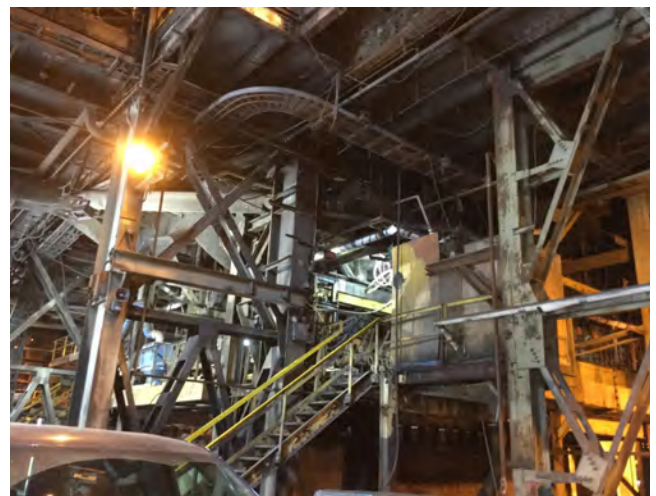
Photo #6: Bottom level of the Furnace Building.
