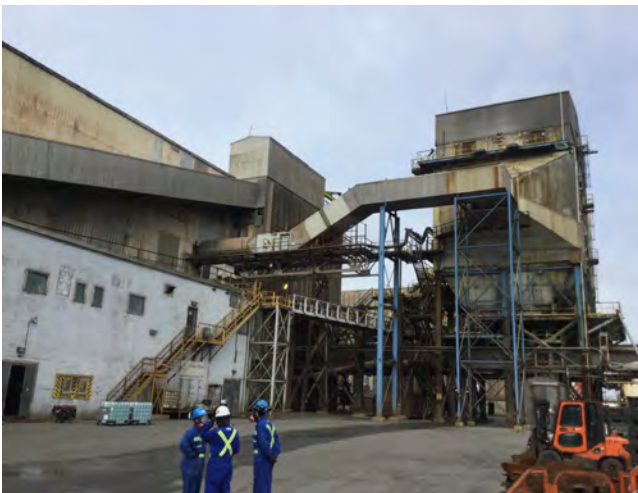
Photo #29: View of the HESP and Sinter Building.
