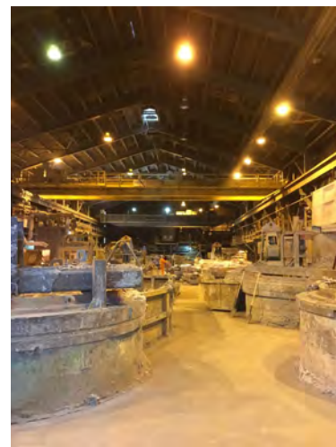
Photo #4: Inside view of the Refinery.
