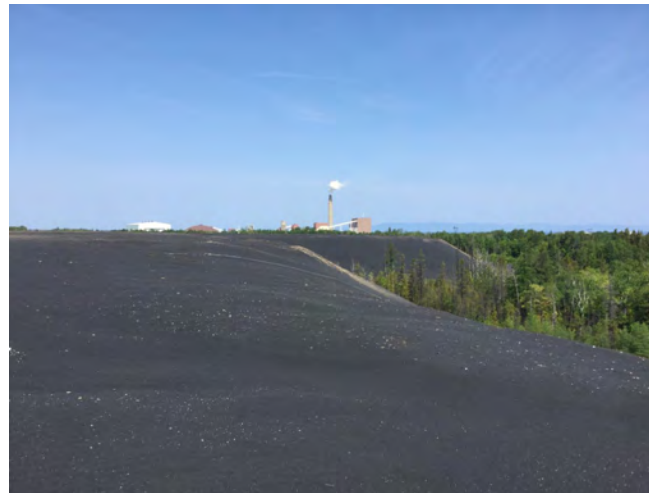
Photo #40: View of the New Slag Pile.
