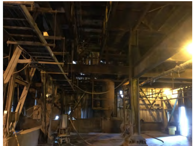
Photo #16: View of the bottom of Charge Preparation Building.
