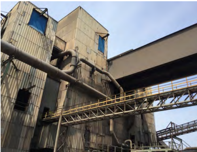
Photo #15: View of the Charge Preparation Building.
