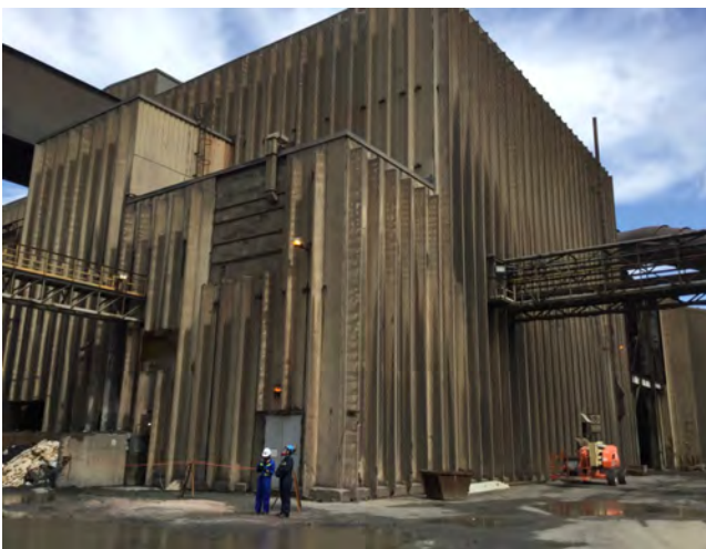
Photo #5: View of the Furnace Building.
