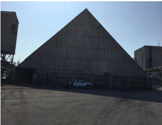
Photo #45: View of the DAP Storage Building.
