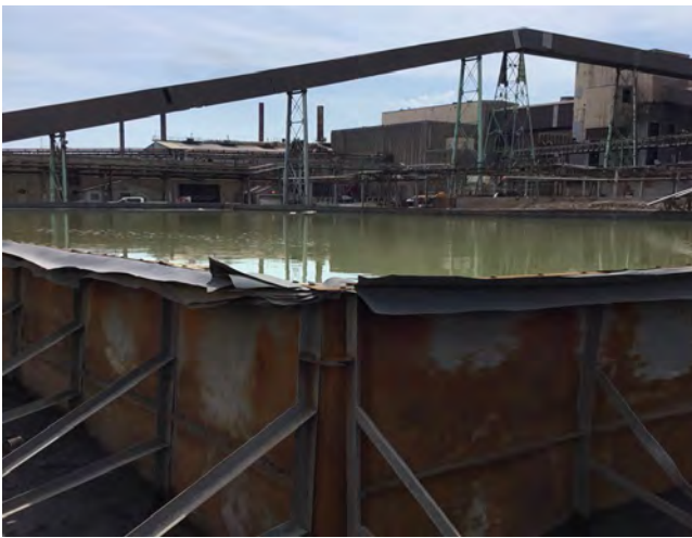
Photo #33: View of the RPW Pool.
