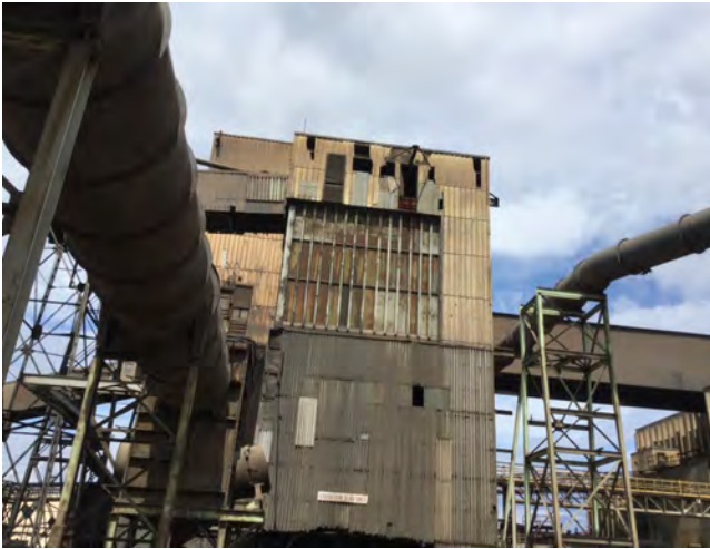
Photo #13: Exterior view of the Crusher Building.
