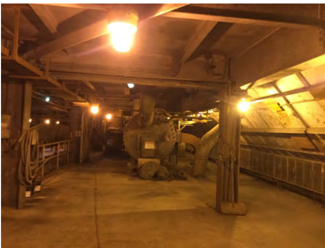
Photo #9: View of underneath Sinter Plant.
