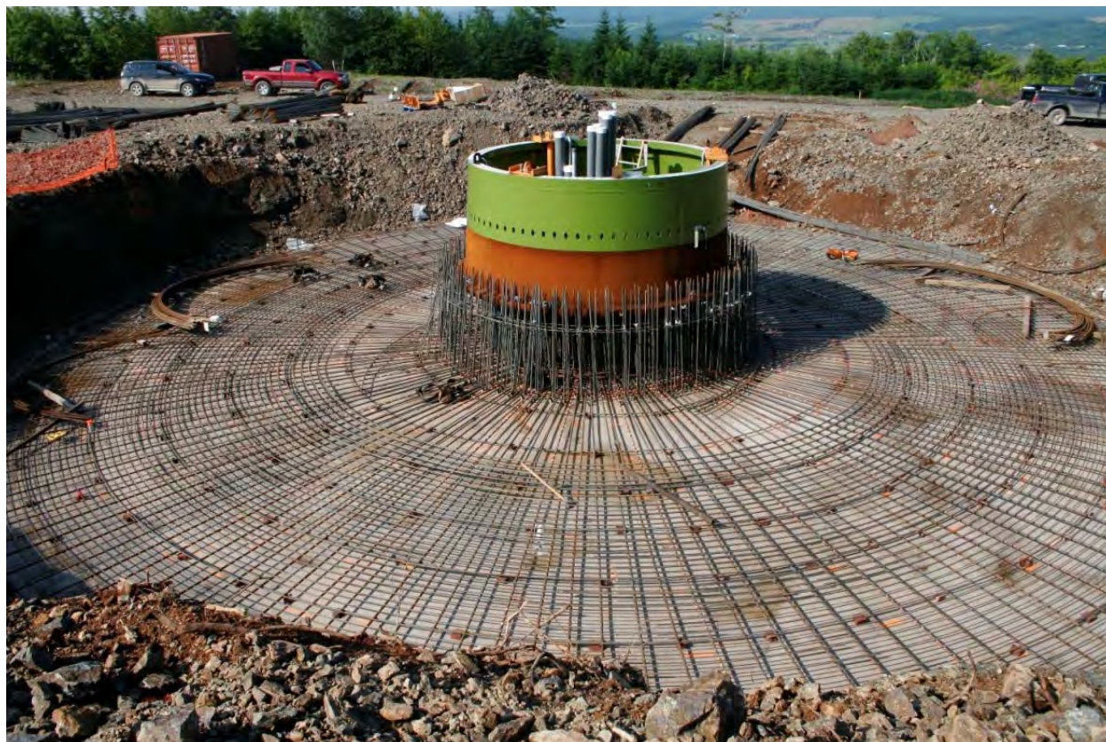
Figure 2-4: Construction of a concrete foundation at Natural Forces’ Fairmount Wind Farm.
