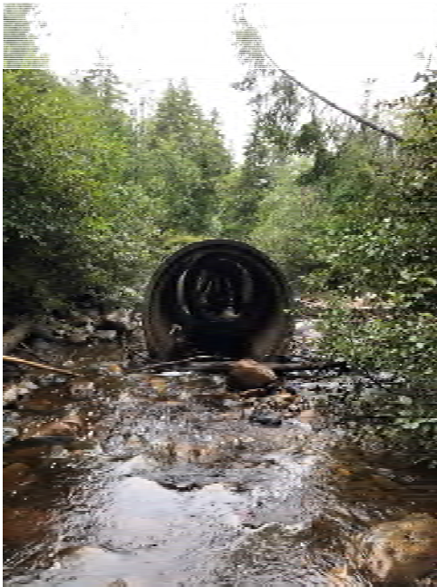
Washed out crossing on BB along the water pipeline that extends from Spruce Lake to Coleson Cove.
