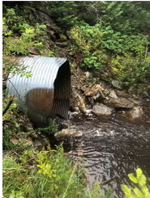
Washed out crossing on BB along the water pipeline that extends from Spruce Lake to Coleson Cove.
