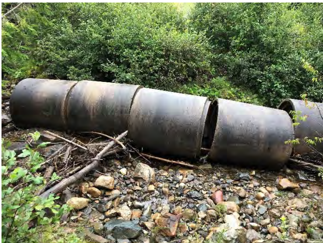
Washed out crossing on BB along the water pipeline that extends from Spruce Lake to Coleson Cove.
