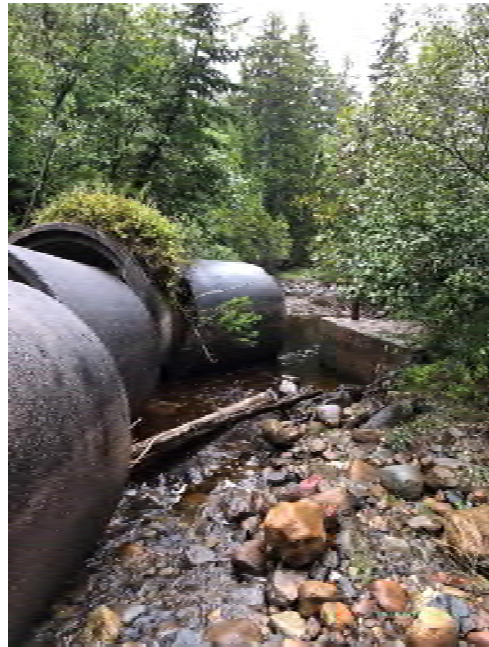
Washed out crossing on BB along the water pipeline that extends from Spruce Lake to Coleson Cove.
