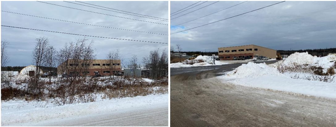
Figure 1: The Simpson Truck and Tractor Parts building (receptor E).
