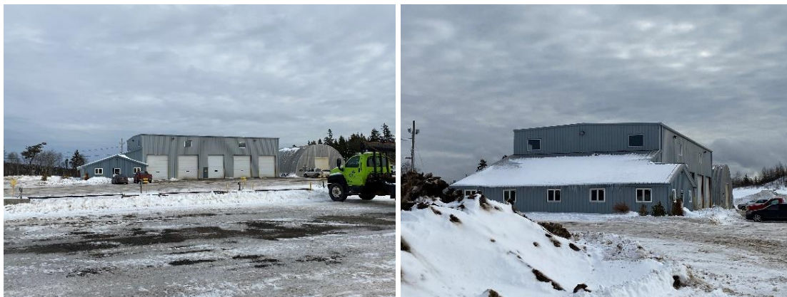
Figure 2: The GFL Environmental building (receptor F).
