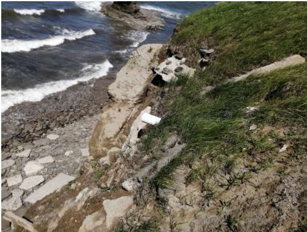
Photo No. 5: Existing Effluent Discharge Pipe (Grow-out Building)
