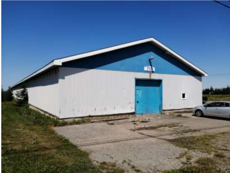
Photo No. 1: Existing Building at 710 rue de l'Acadie
