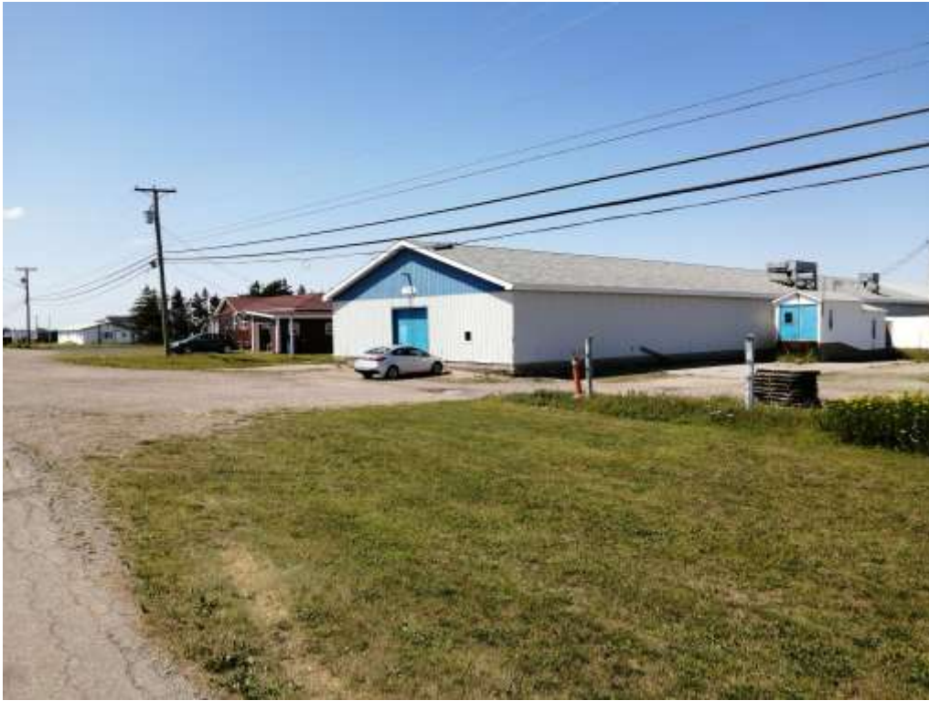
Photo No. 1: Hatchery Building and Site Entrance West
