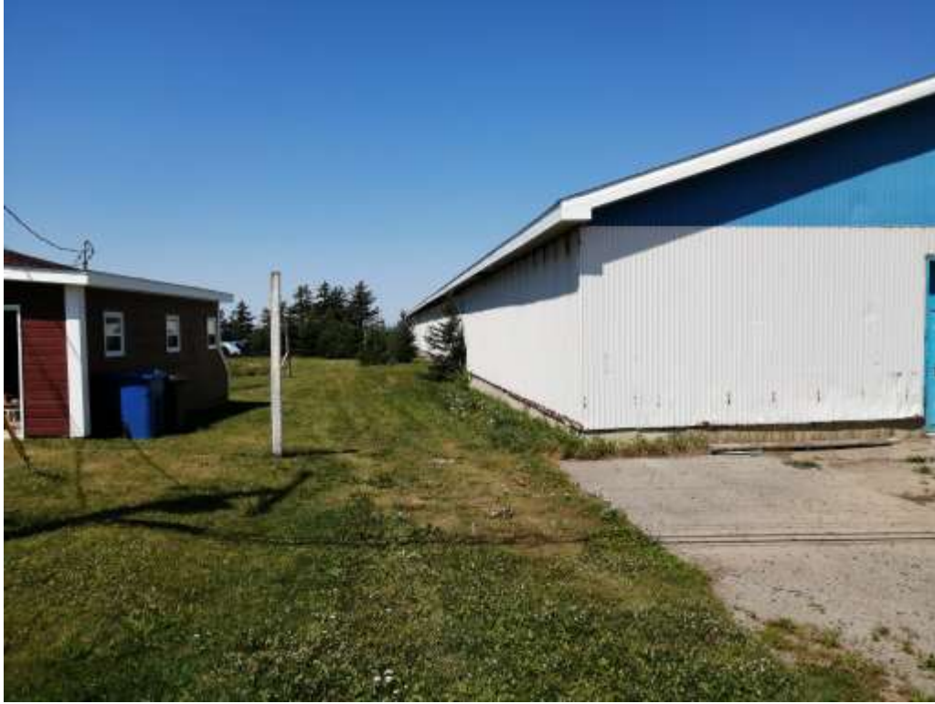
Photo No. 3: West Side of Hatchery Building and Home (left)
