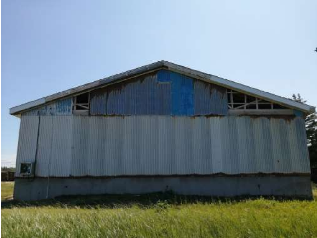
Photo No. 2: Rear of Hatchery Building
