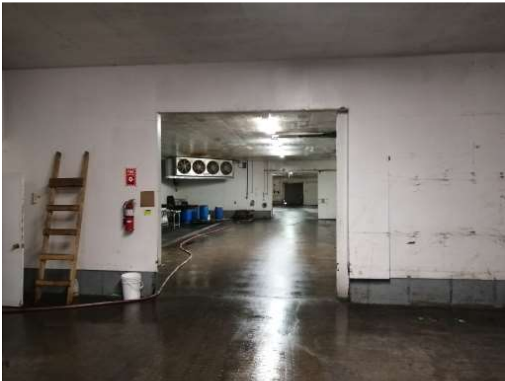
Photo No. 4: Building Interior
