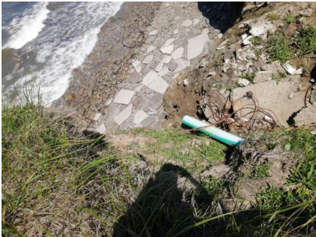
Photo No. 8: Freshwater Hatchery Existing Outfall Pipe
