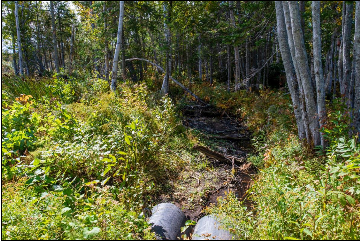
Figure 6: At the stream, south of the turbine, facing north-east.
