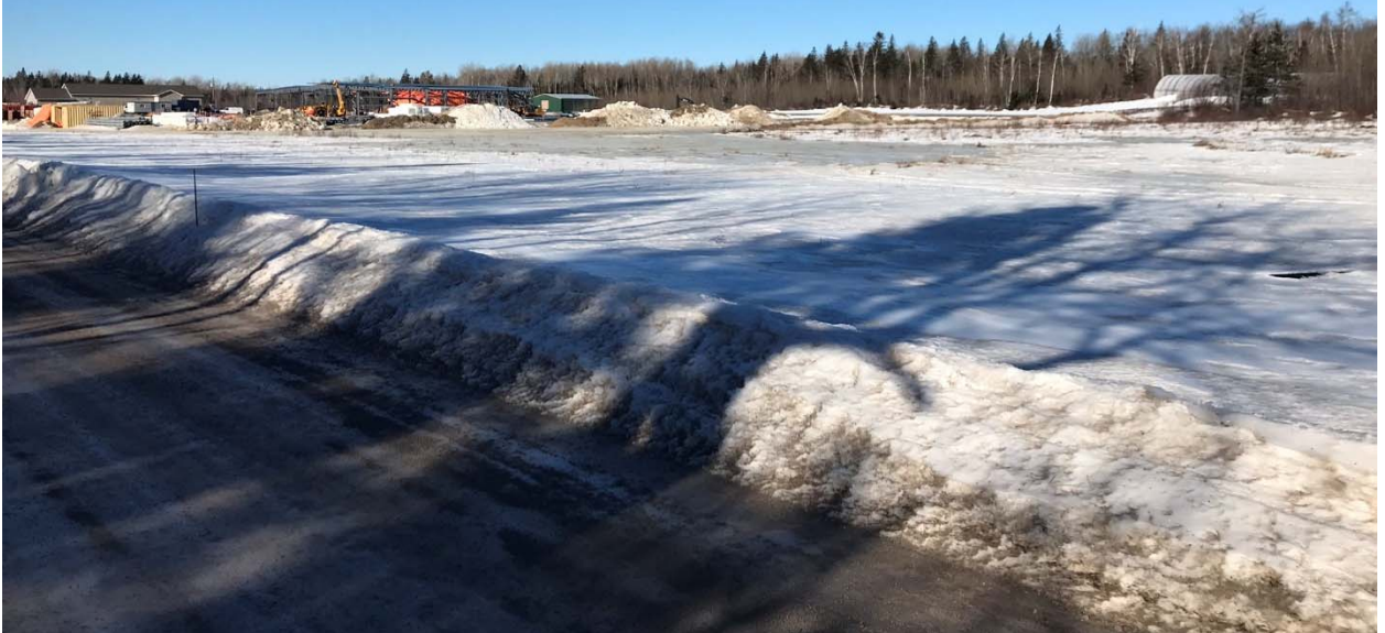
Construction of the Agricultural Building well underway.
