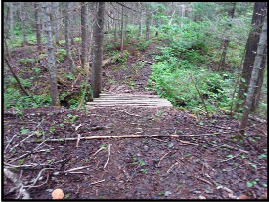
Photo 1: Existing wooden bridge on Trail E/Trail H at Watercourse 2 crossing location.
