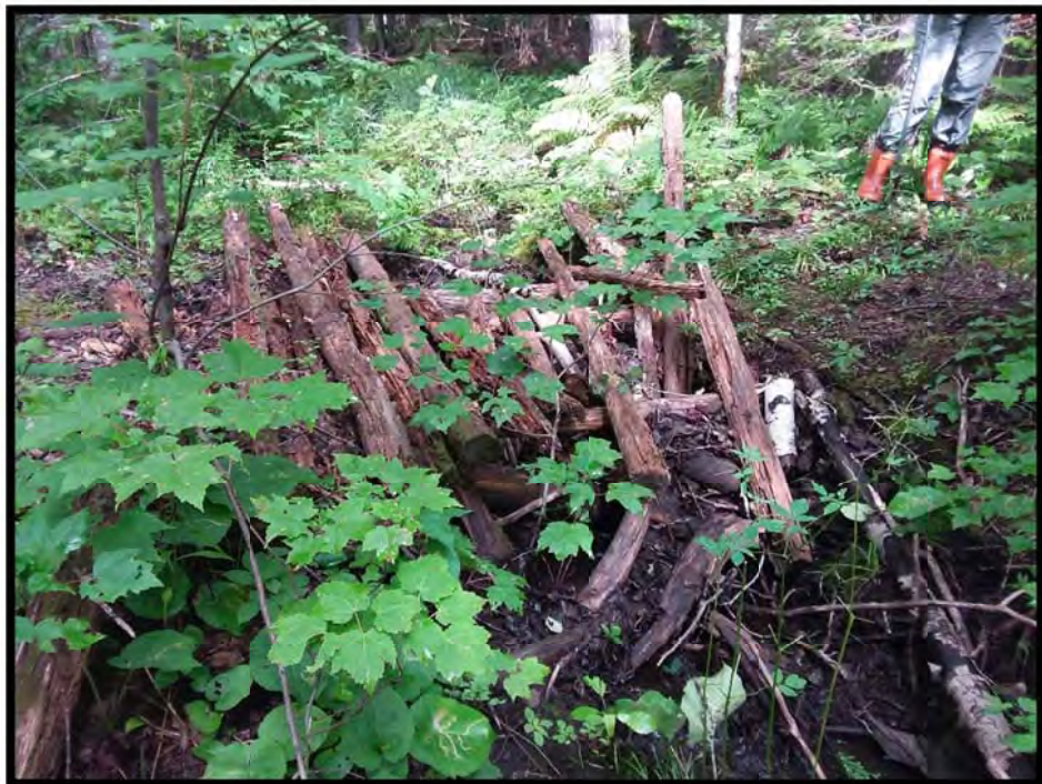
Photo 2: Existing wooden bridge on Trail F at Watercourse 3 crossing location.
