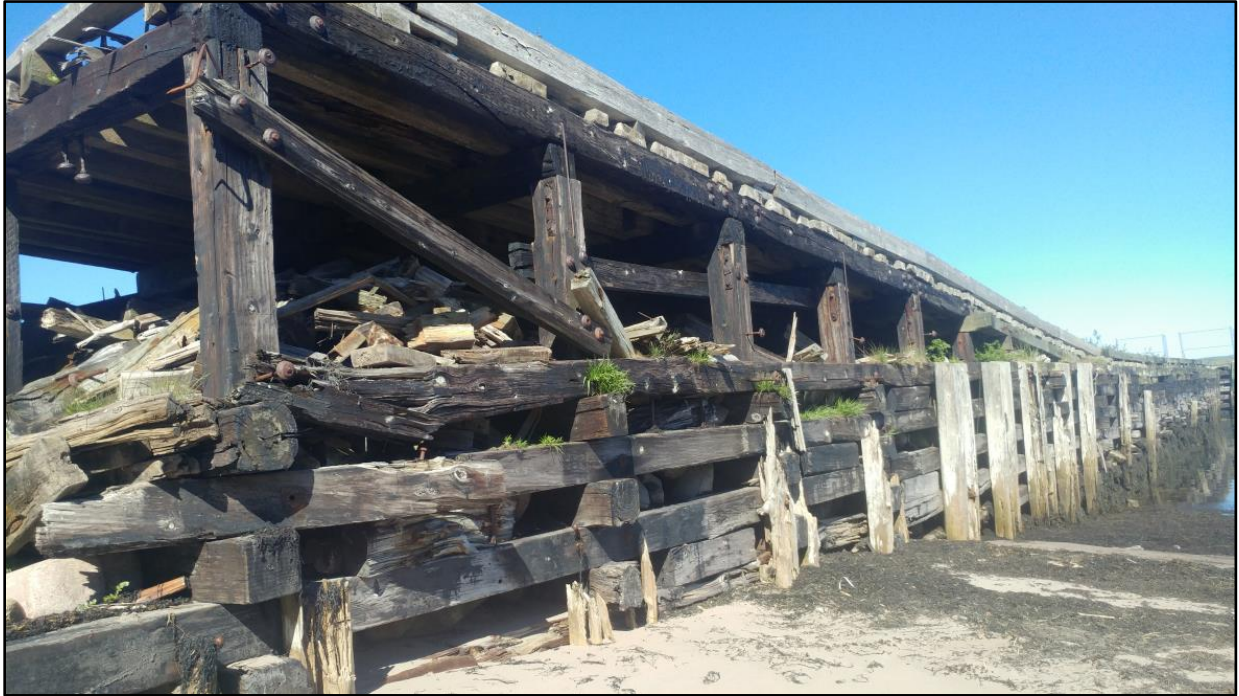
Photo 7: Maces Bay DFO-SCH wharf structure looking northwest (June 22, 2018).
