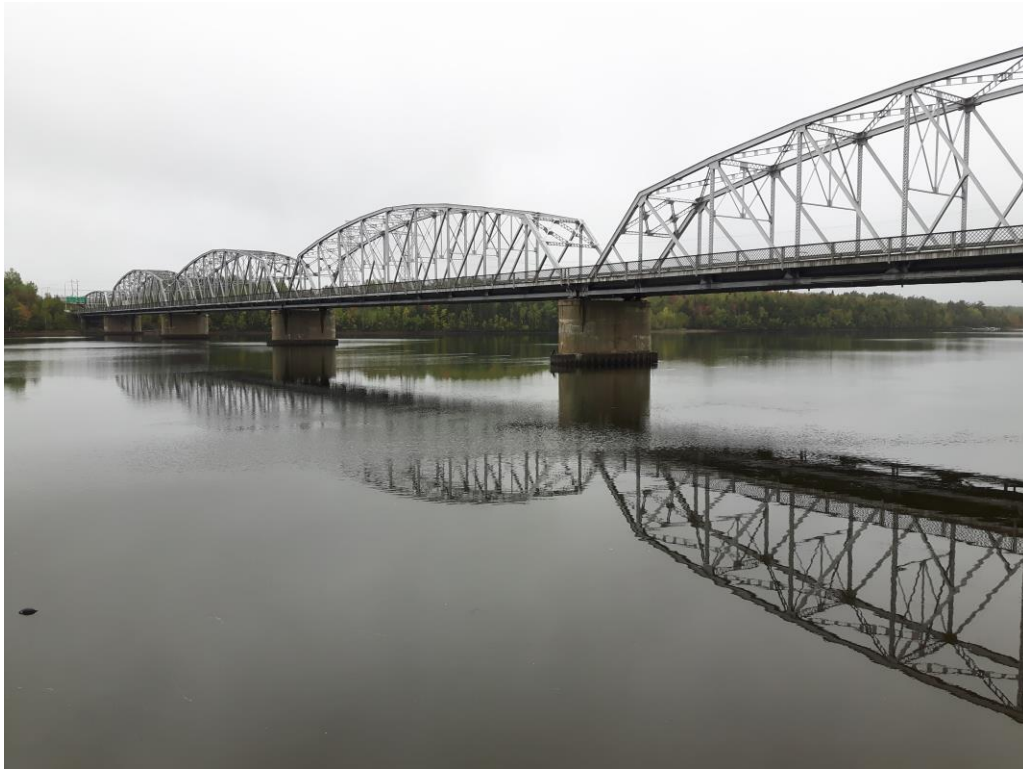
Photo 2: View of the existing bridge, facing south (September 27, 2017).
