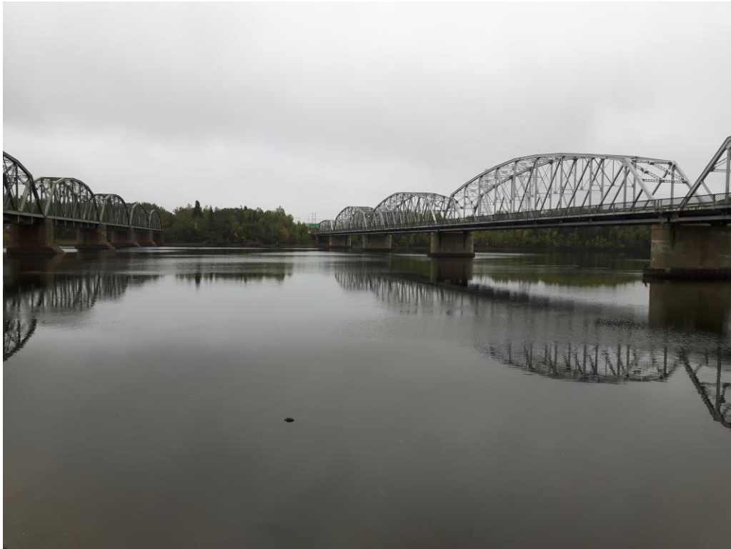
Photo 3: View of the existing bridge (right) and the rail bridge (left) (September 27, 2017).
