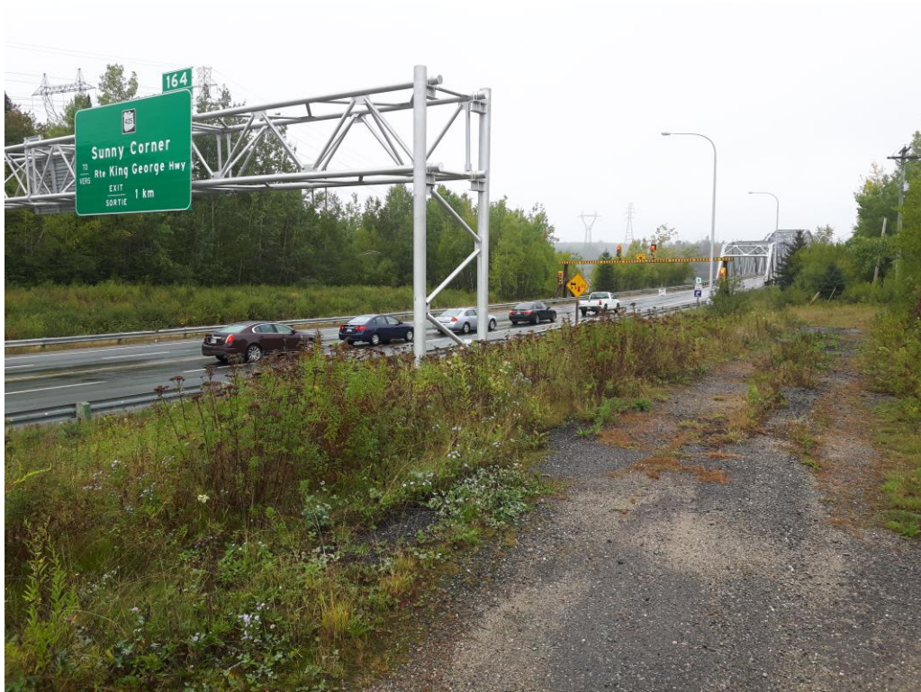
Photo 4: View of Route 8, south of the existing bridge, facing northwest (September 27, 2017).
