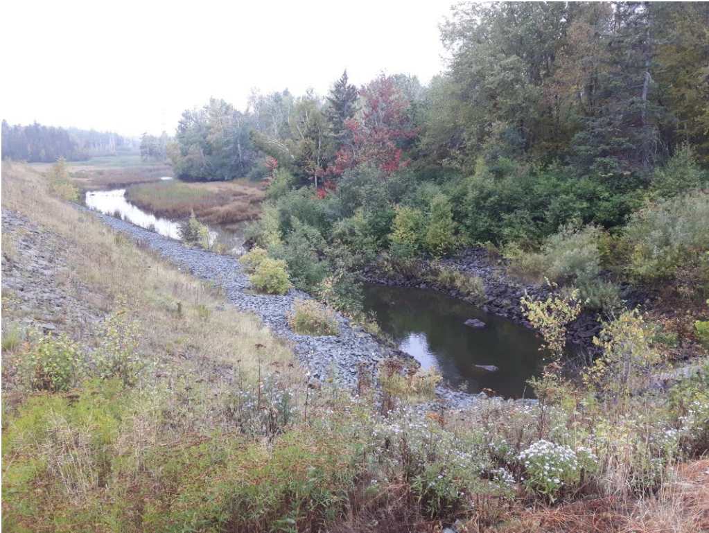
Photo 8: View of Oxford Brook on PID 40437139, facing south (September 27, 2017).
