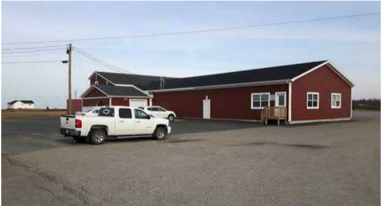
Photo No. 1: Existing Fish Plant Looking North
