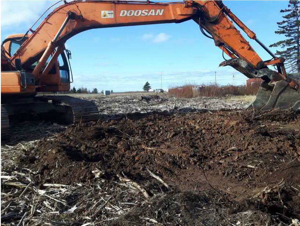
Backfilling TP17-04 following the investigation at this location.
