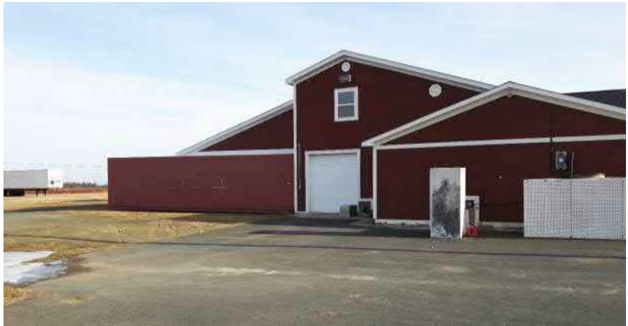
Photo No. 2: Existing Fish Plant Looking East
