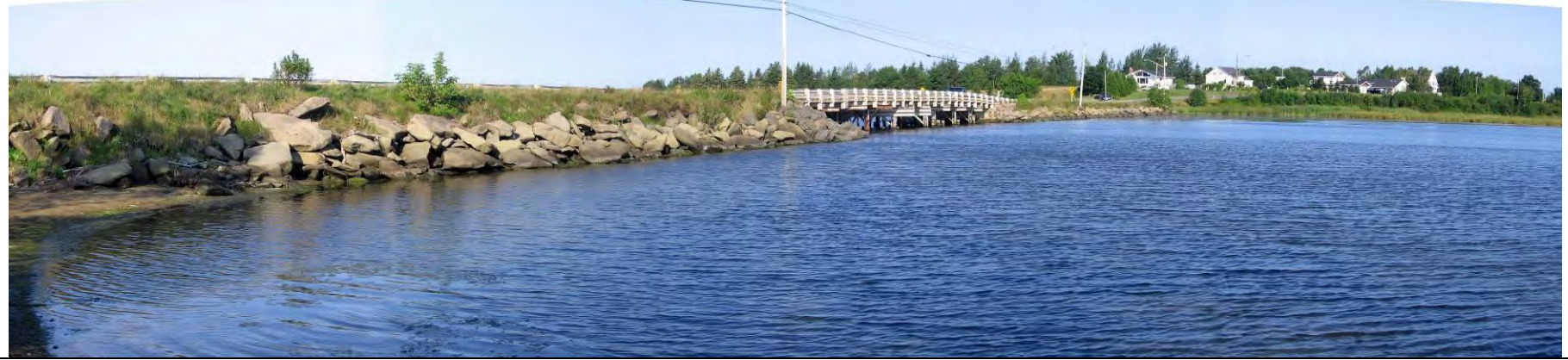
Photograph 1 Right of Way showing causeway and bridge structure facing west
