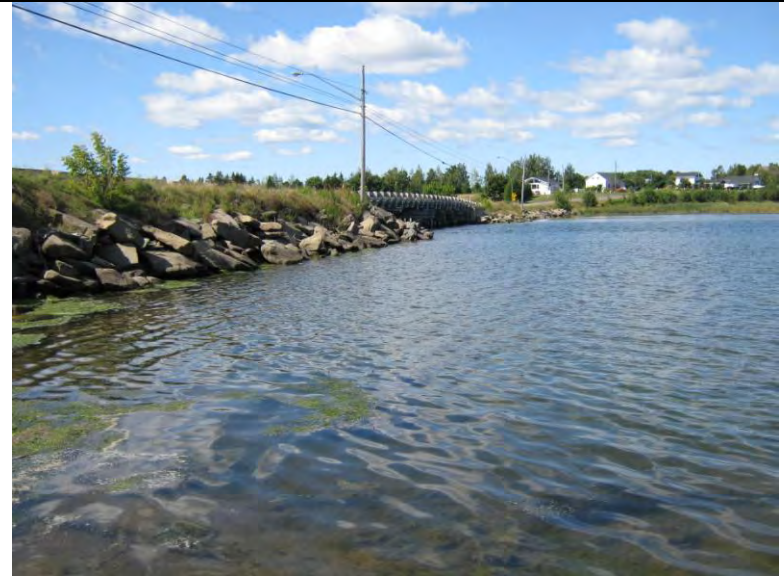
Photograph 4 Existing bridge and causeway facing west
