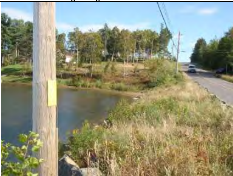
Photo 5 shoreline on downstream side of existing bridge
