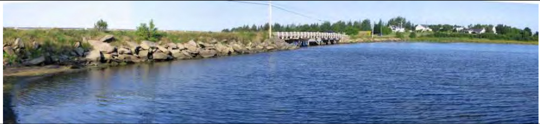
Photo 1 Right of Way showing causeway and bridge structure downstream
