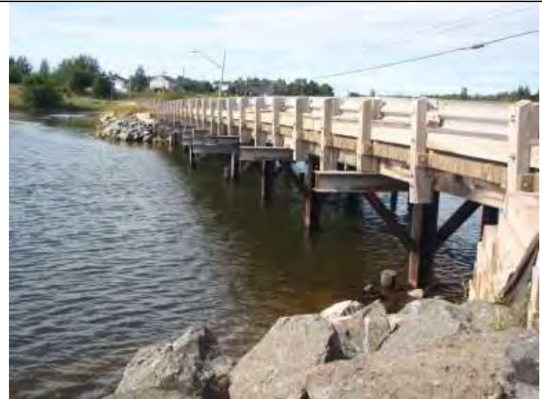
Photo 4 Existing bridge structure
