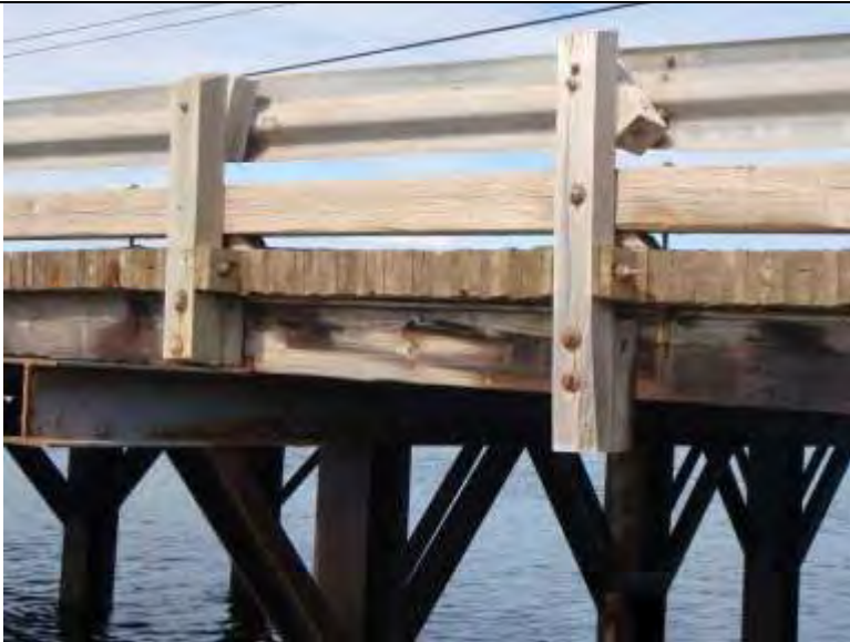
Photo 3 Existing bridge structure
