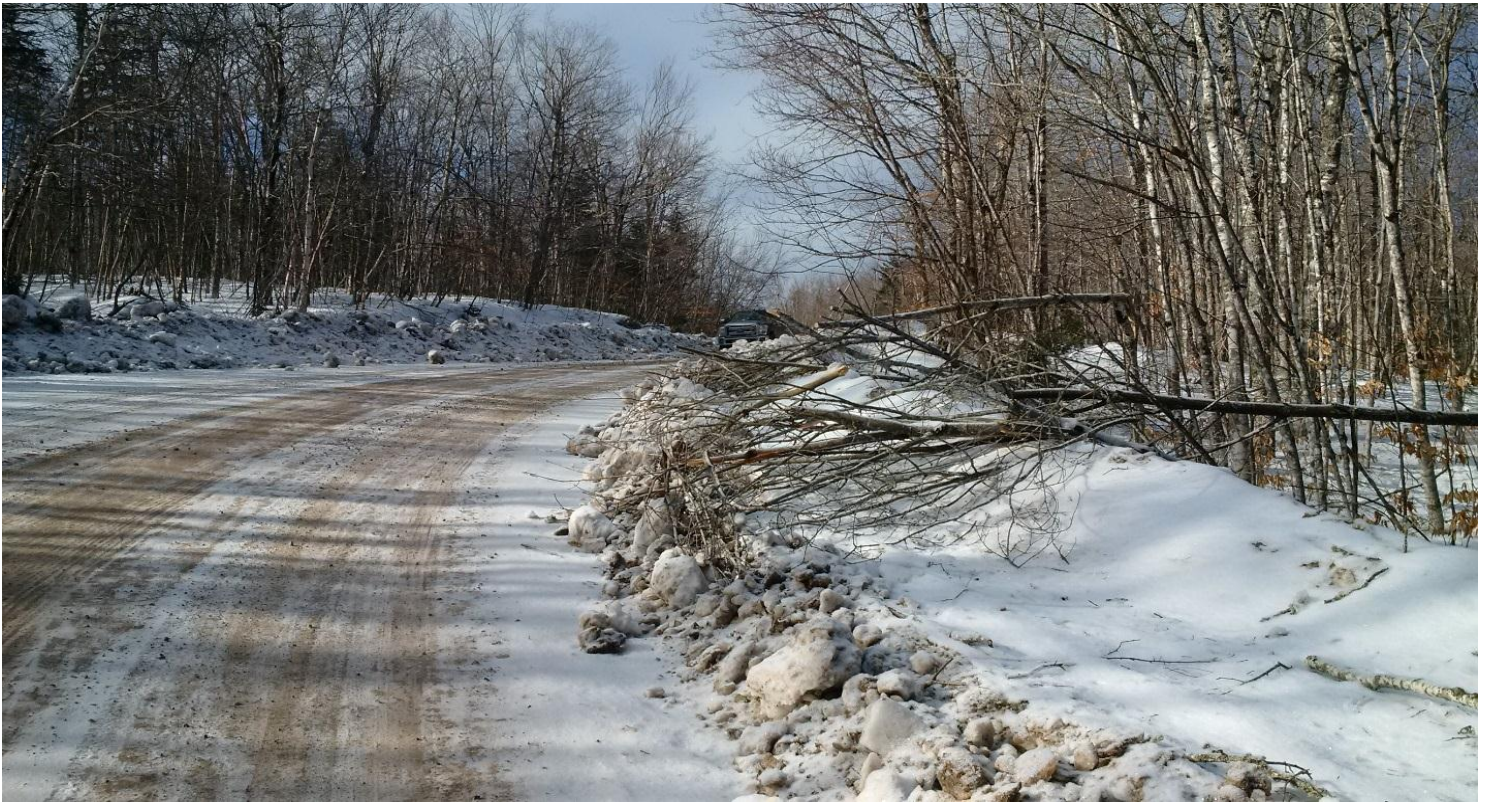
17- Prosser Brook Hill -Pull Truck Required on Hill +16% Grade - Also trees to trim back
