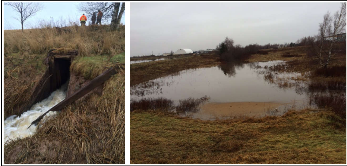
Figure 2: Photos of PSW at Existing Aboiteau Structure
