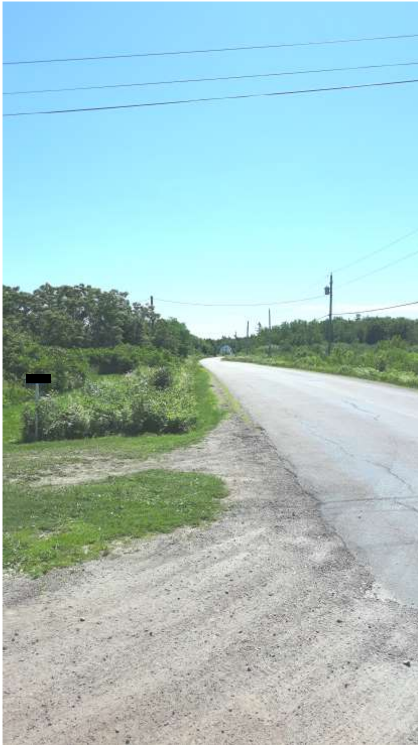
Photo No. 10: Route 955 Looking East from Campground Entrance
