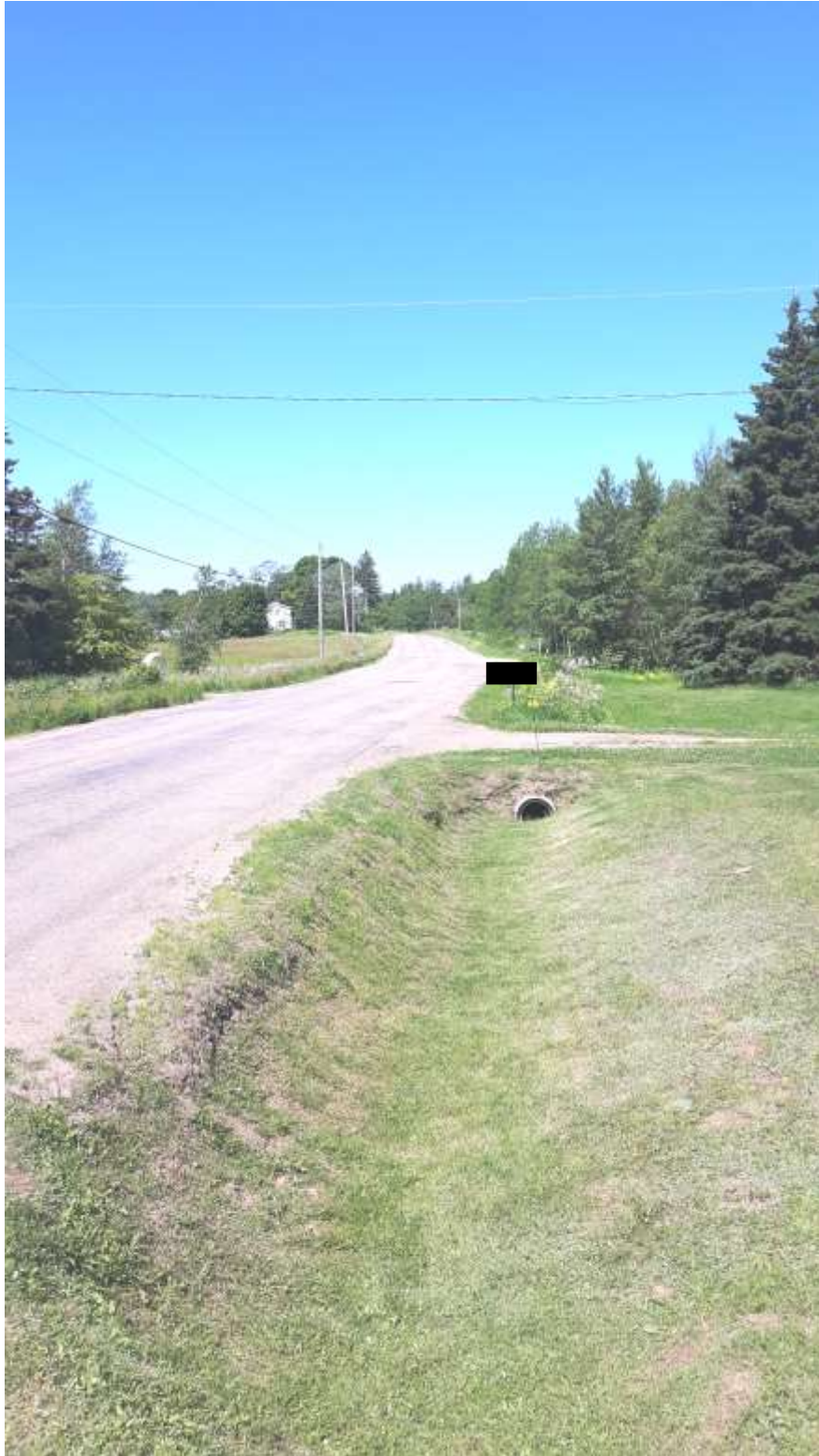
Photo No. 9: Route 955 Looking West from Campground Entrance
