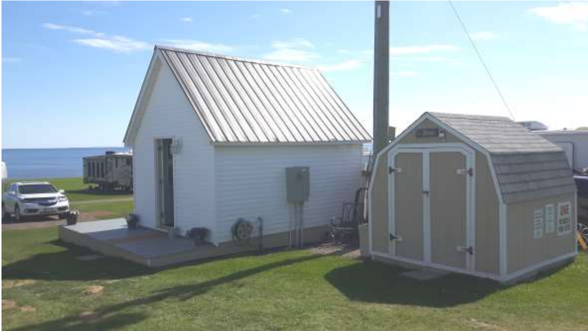
Photo No. 3: Well Pumphouse (Left) and Shed
