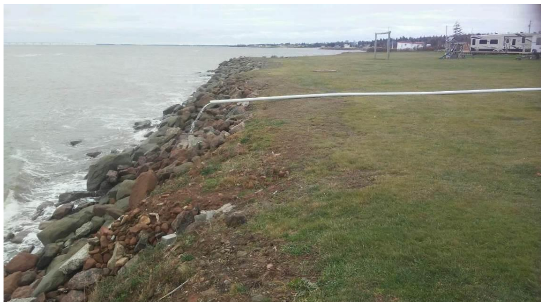
Photo 5: View of water discharge (November 19, 2017)
