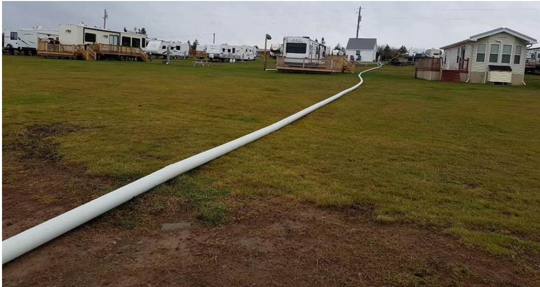
Photo 4: View of water discharge line directing pumped water towards the Northumberland Strait (November 19, 2017).
