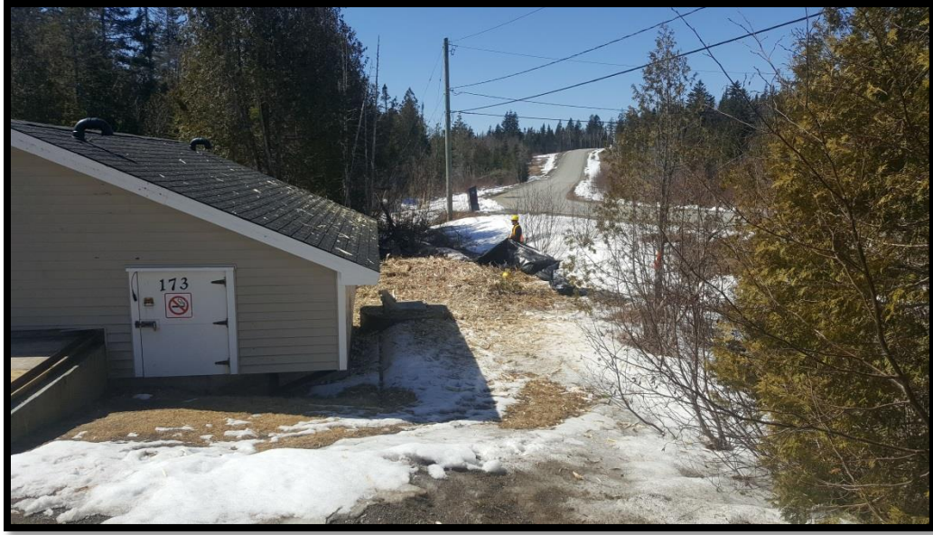
Photo 1: Looking west towards the WWTF building and Secord Street.
