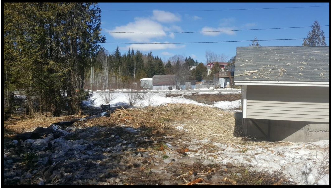
Photo 3: Looking northwest during clearing activities.
