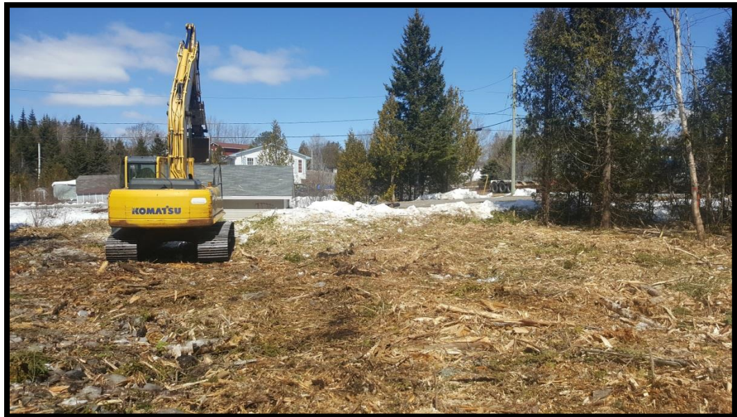
Photo 4: Looking north/northwest during clearing activities.
