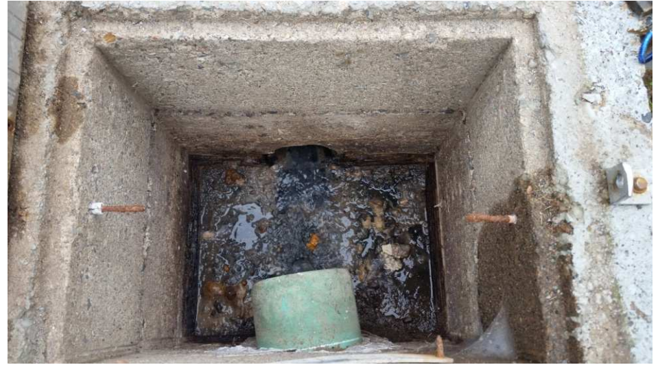
Inside inlet box
