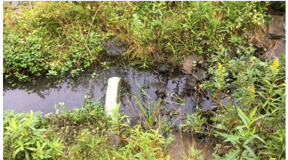
Outfall in ditch along Secord Street
