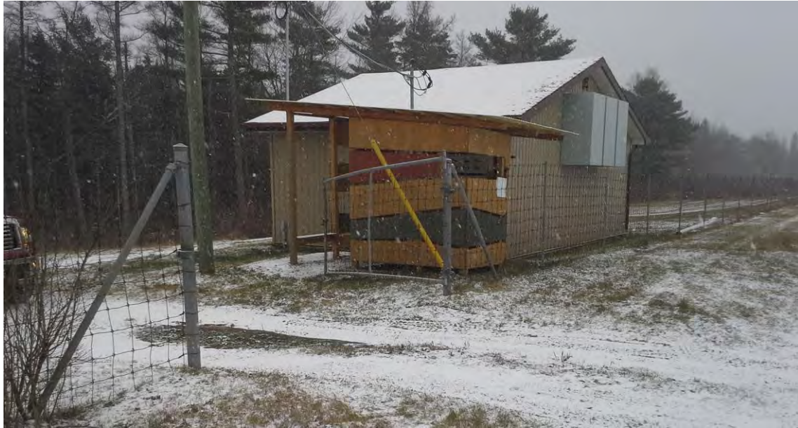
Photo No. 3: Security Gate, Bird Watching Platform and Blower Building (December, 2016)
