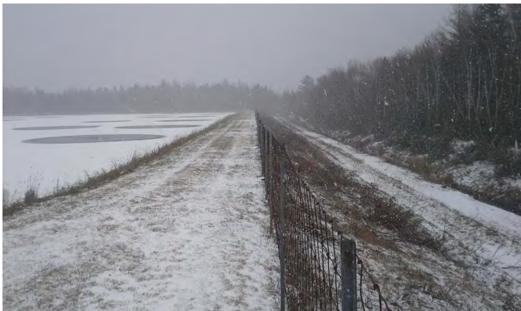
Photo No. 5: Lagoon Grassed Area (December 2016)
