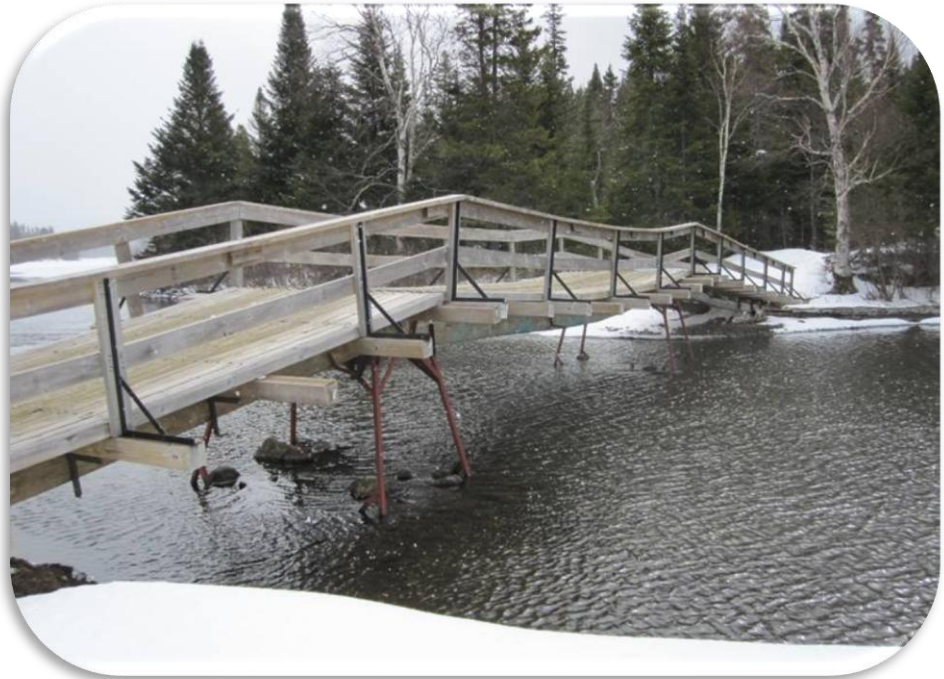
Photo 10: Existing Bridge over Bathurst Lake near Bathurst Camps
