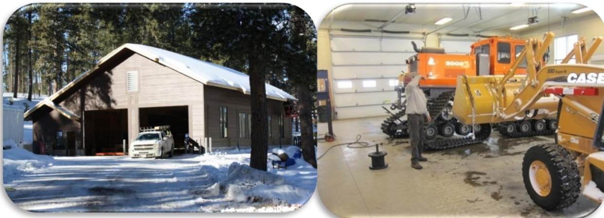
Photos 25 and 26: Exterior (left) and interior (right) views of new Black Hills shop built in 2010
