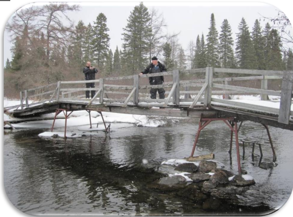
Photo 11: Existing Bridge over Moose Creek
