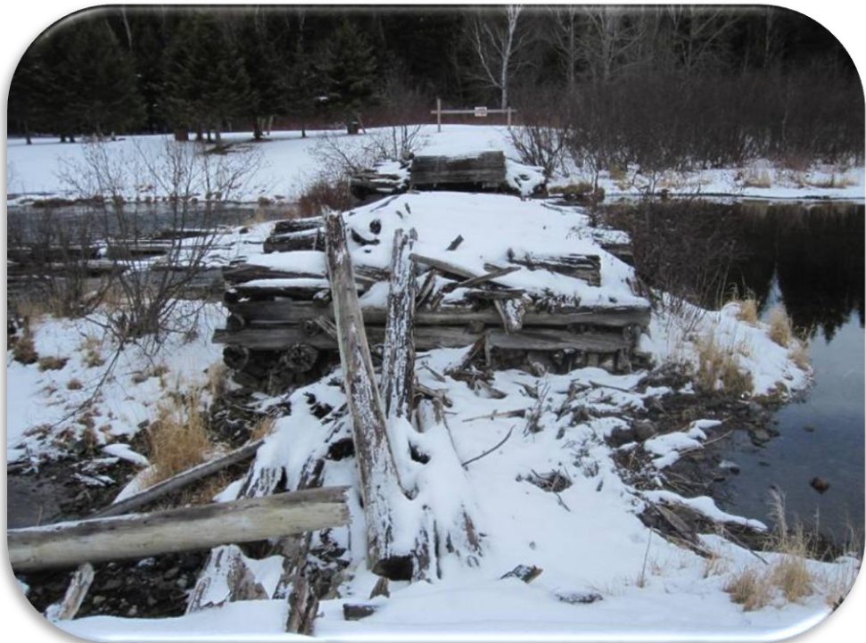
Photo 9: Existing remnants of old bridge over Armstrong Brook
