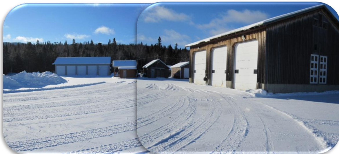
Photos 20 & 21: Existing cold storage (left) and heated shop (right) buildings at Mt. Carleton Park
