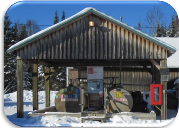
Photo 27: Existing Mt. Carleton fuel depot area
