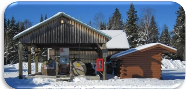
Photo 37: Existing Mt. Carleton fuel depot area
