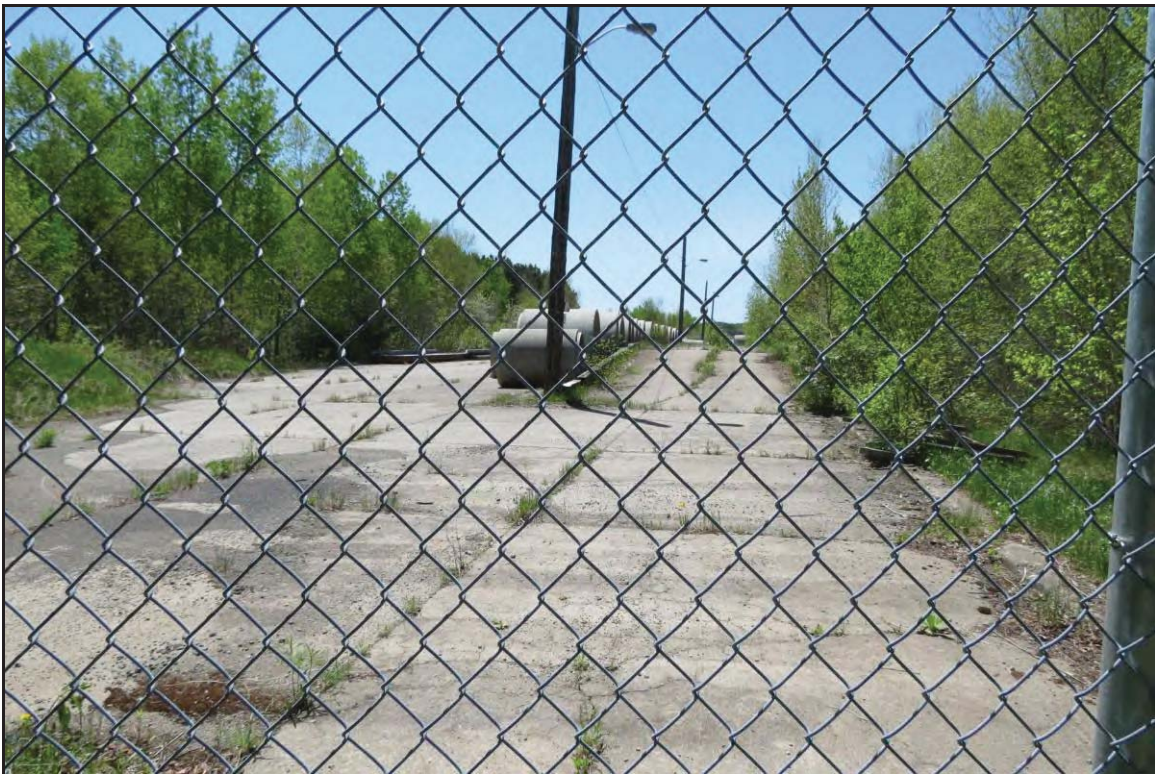
PLATE 5: Storage area in Section Two; facing west; May 29, 2014.
