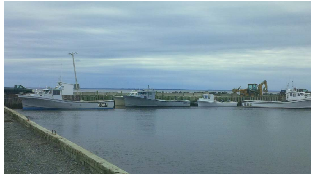
Wharf where the water level was monitored
