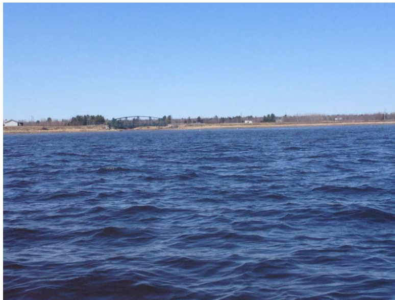
Bridge seen from further away
