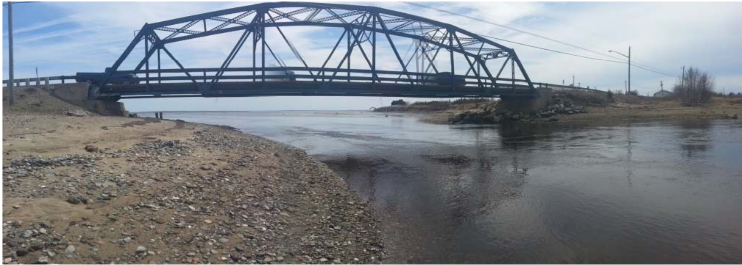
Bridge on MicMac Road
