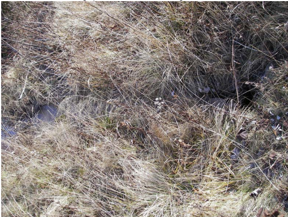
Photo 12: Watercourse 4 – Looking upstream from culvert along access road
