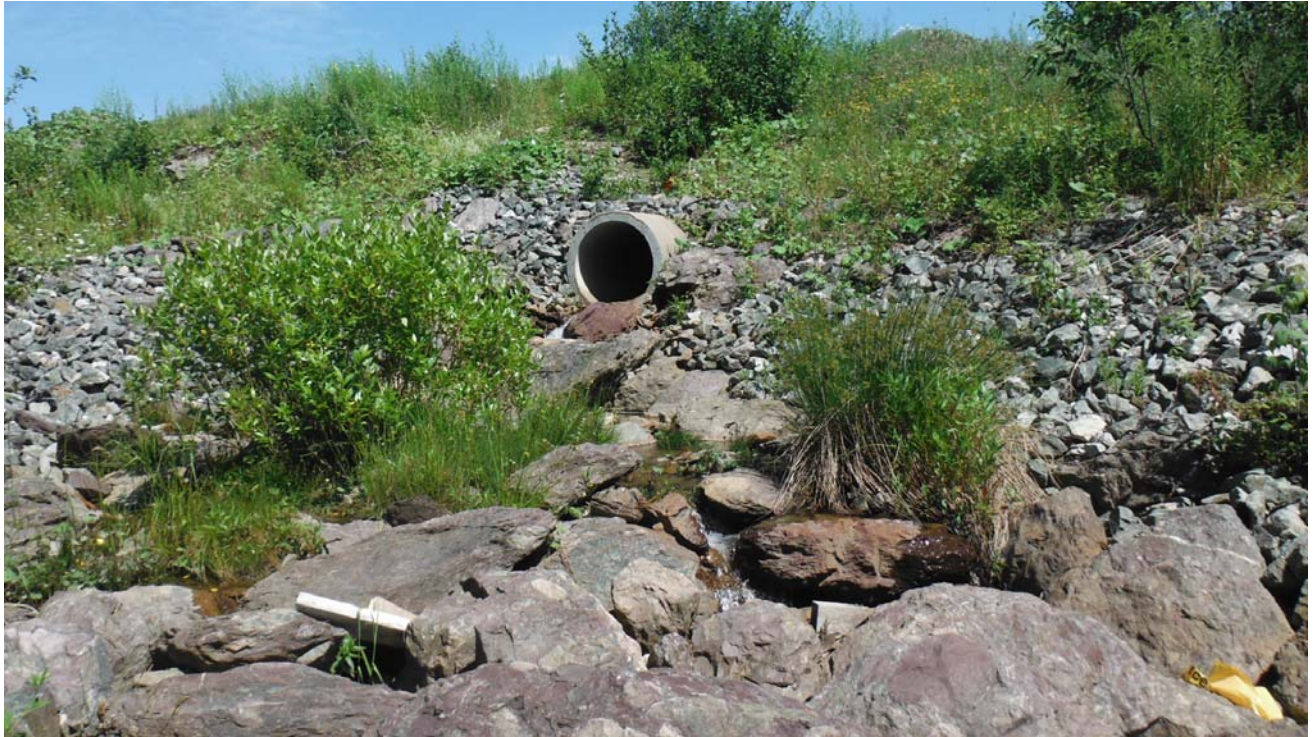
Photo 1: Watercourse 1 – Culvert under McIlveen Drive that feeds watercourse
