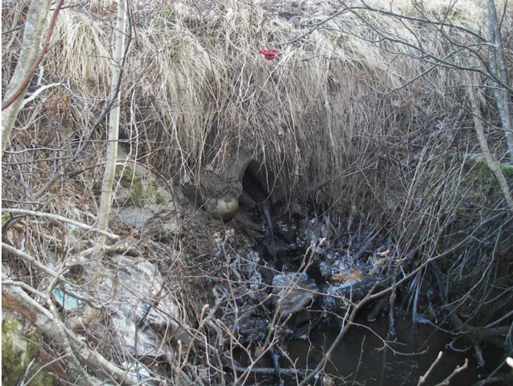
Photo 13: Watercourse 4 – Looking at culvert from downstream
