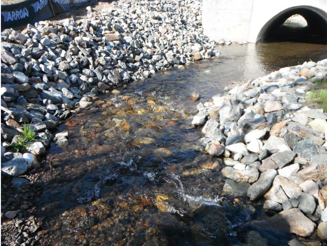
Photo 7: Watercourse 2 – Immediately upstream of culvert under Whitebone Way
