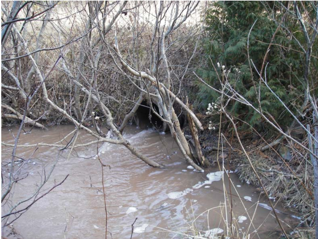
Photo 15: Watercourse 5 – Looking at culvert from downstream
