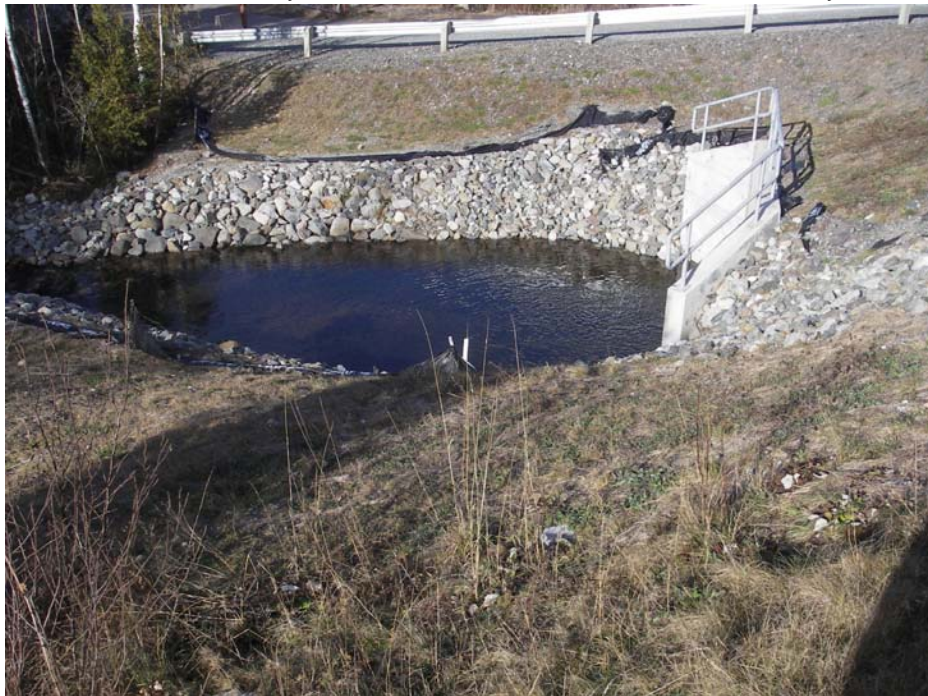
Photo 8: Watercourse 2 – Immediately downstream of culvert under Whitebone Way
