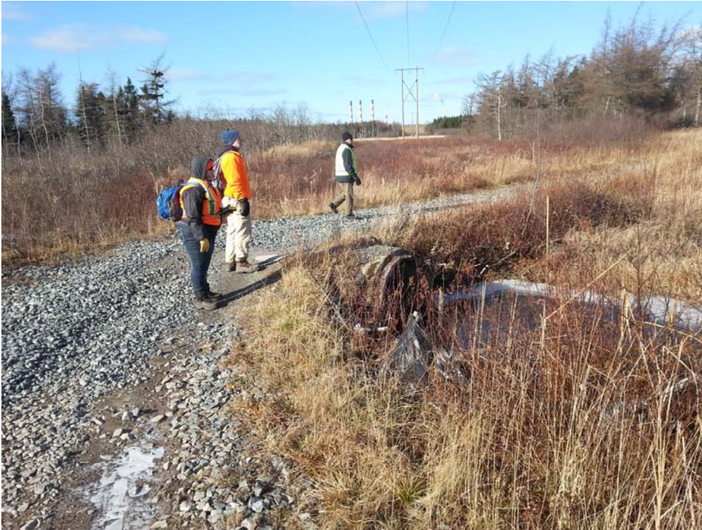
Photo 17: Watercourse 6 – Looking northwest at culvert of access road
