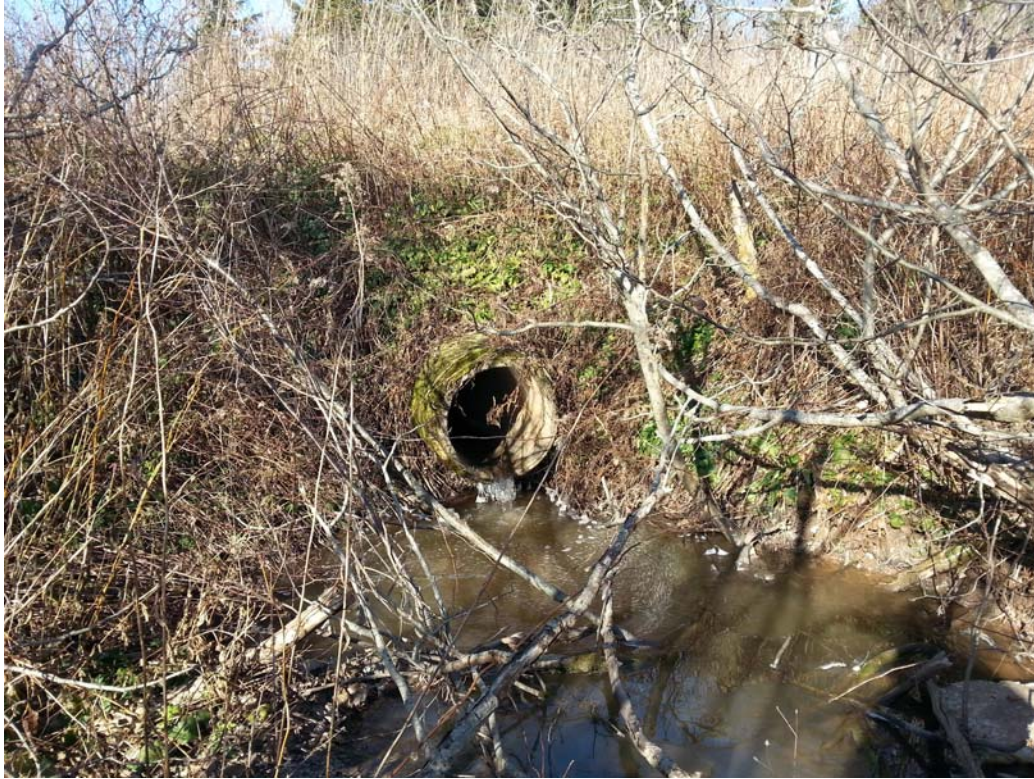
Photo 29: Watercourse 11 – Looking at culvert from downstream
