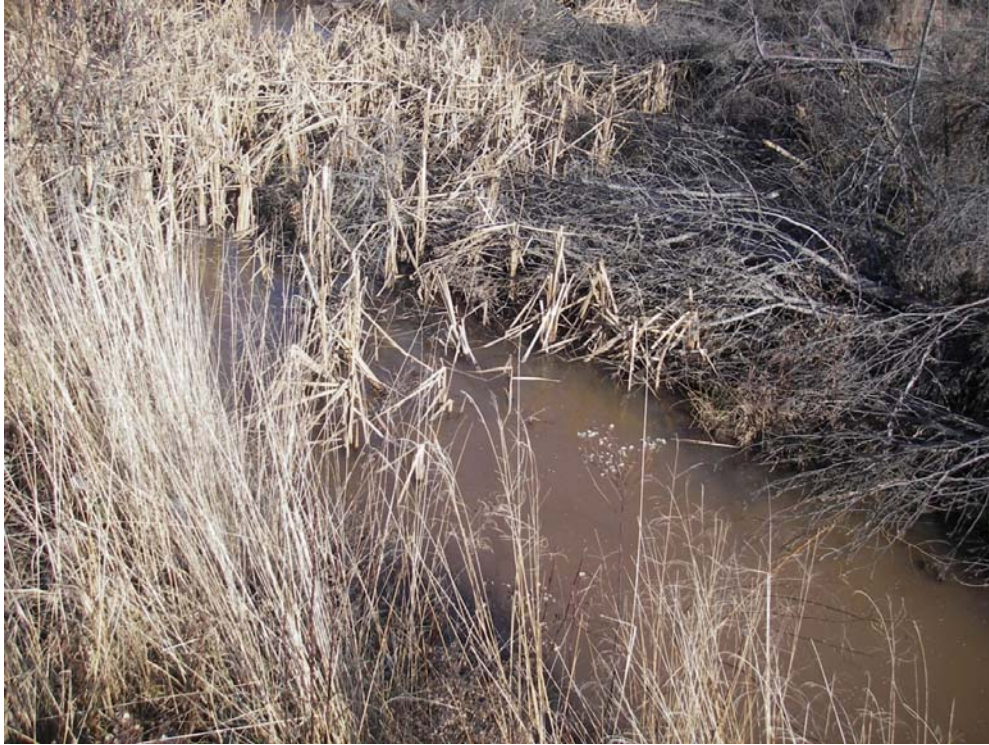
Photo 9: Watercourse 3 – Looking upstream from culvert along access road
