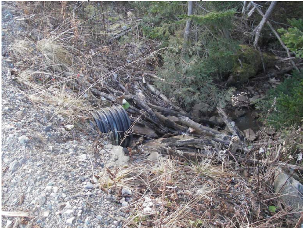
Photo 10: Watercourse 3 – Looking downstream from culvert along access road
