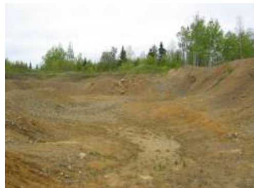
Stop 6 - Clay-rich basal till and weathered bedrock in borrow pit near the Restigouche Mine.
