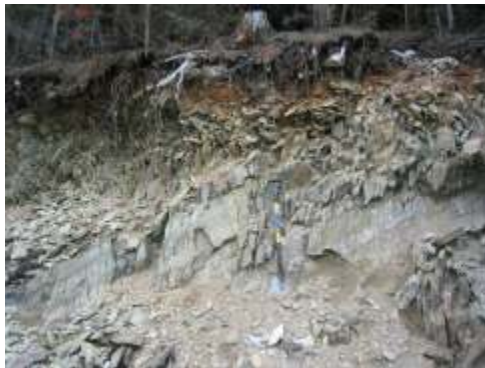
Stop 23 - Thin till and a veneer of broken rock over Temiscouata Formation sedimentary rocks. Note downslope creep (from right to left) in upper parts of the fractured bedrock. This site is at a higher elevation than the previous 10 photographs, and is approximately 1 km to the southeast.
